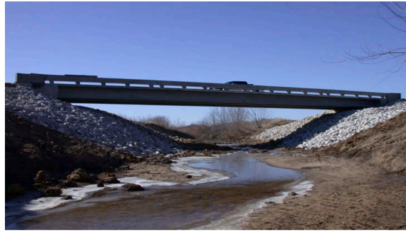
Fig. 2. Mars Hill UHPC bridge in Wapello County, Iowa [55].
