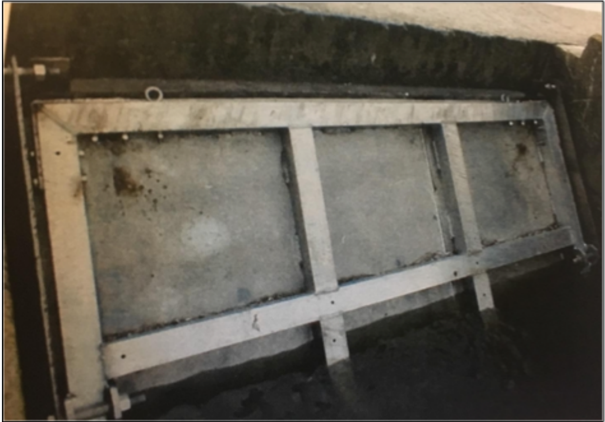
Figure 3. Photograph of a current stainless steel, top-hinged flapgate at Waupoppin Canal, Lake Mattamuskeet, North Carolina (Godwin 2004).
