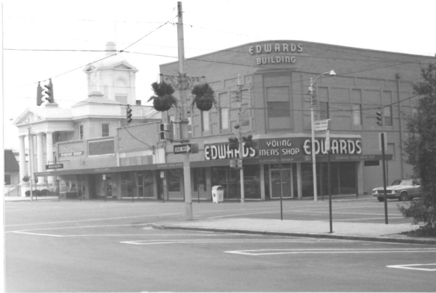
Figure 2. Block number 10 is one of the blocks meeting both of the Central Business Index Method indices. This block has a CBHI of 1.00 and a CBII of 80 percent.
