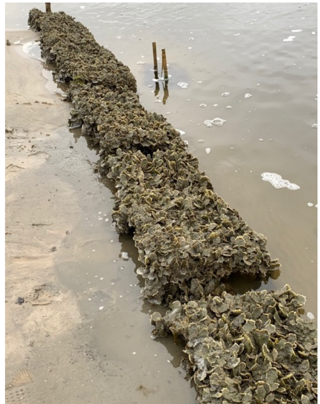
Figure 2. Low-relief Oyster Catcher™ reef 7 months post-construction (Site 4, February 2021). Photo credit: Nina Woodard
