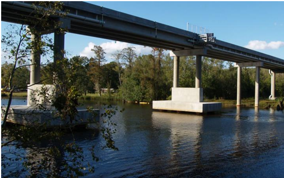
Figure 24. View of the Grimesland Bridge
