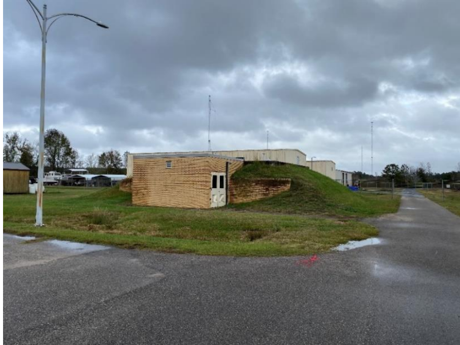
Figure 20. West Water Treatment Building
