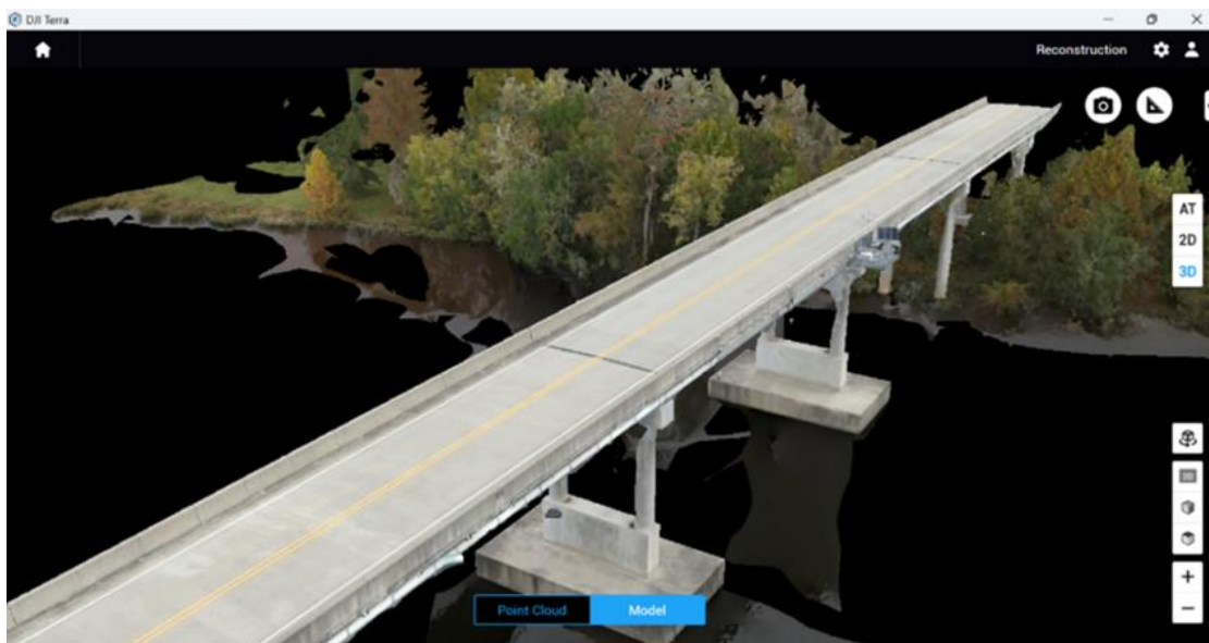
Figure 41. Daylight Photogrammetric Model of the Grimesland Bridge in DJI Terra
