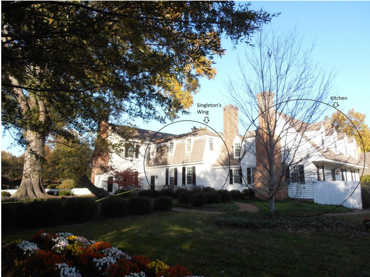
Figure 11: Photograph of Bassett Hall from the garden in the rear of the house. The kitchen wing, added by the Rockefellers, is on the right. The wing added by Singleton is in the middle, and the main/original building is the furthest left in the picture. Photo by author.
