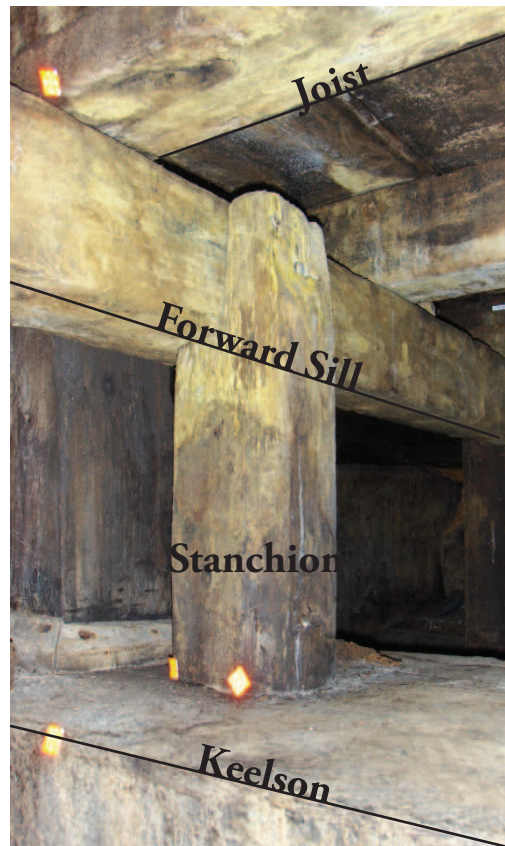
Figure 4-2. The small stanchion atop the keelson, just behind a sill.
