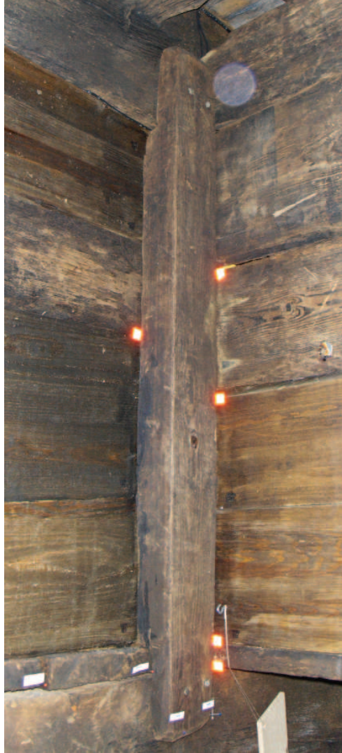
Figure 4-10: The forward starboard smoke bay stanchion.
