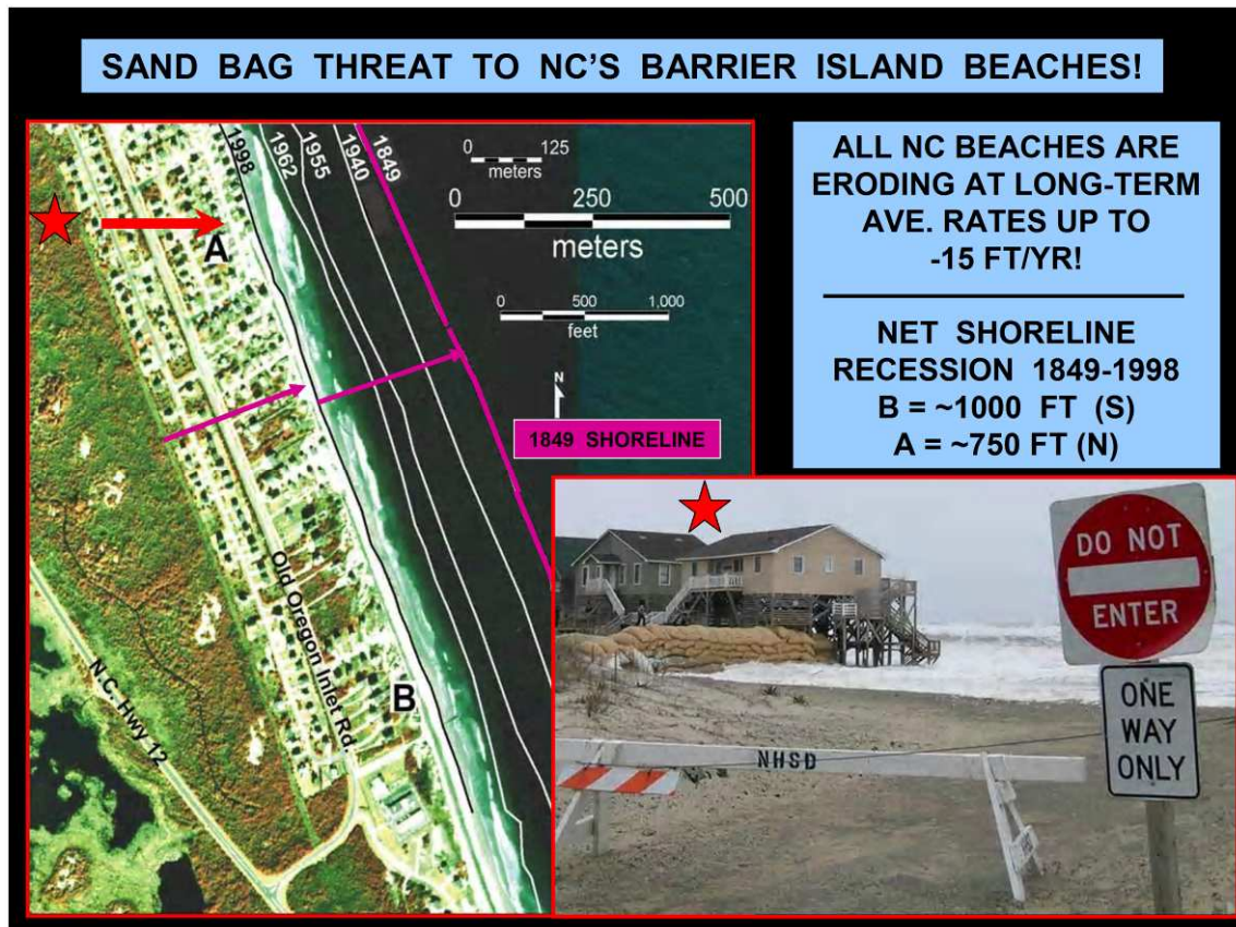
Figure 20. Erosion and sandbag issues at South Nags Head (from Riggs et al., 2008).
