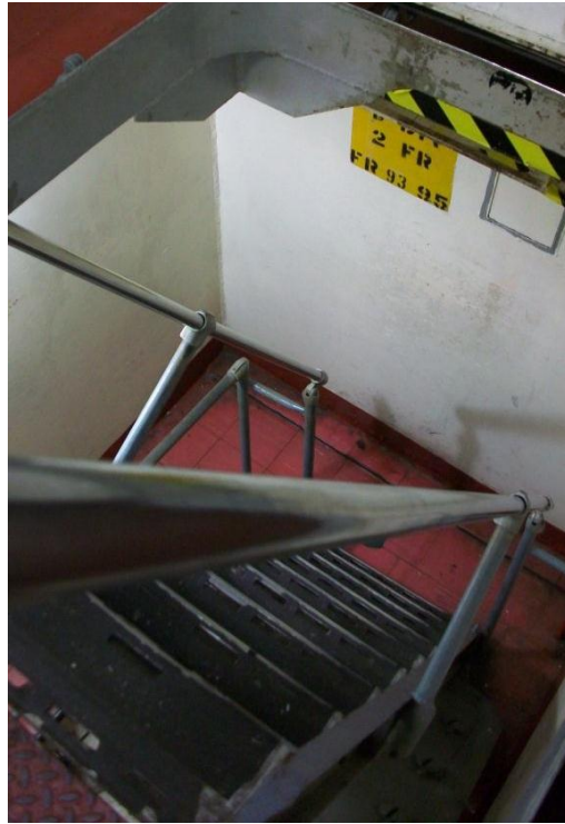
Photograph 36: Ladder on Tour Route 2, descending to one of Yorktown 's engine rooms. This ladder was installed by the museum to make visitor access easier.
