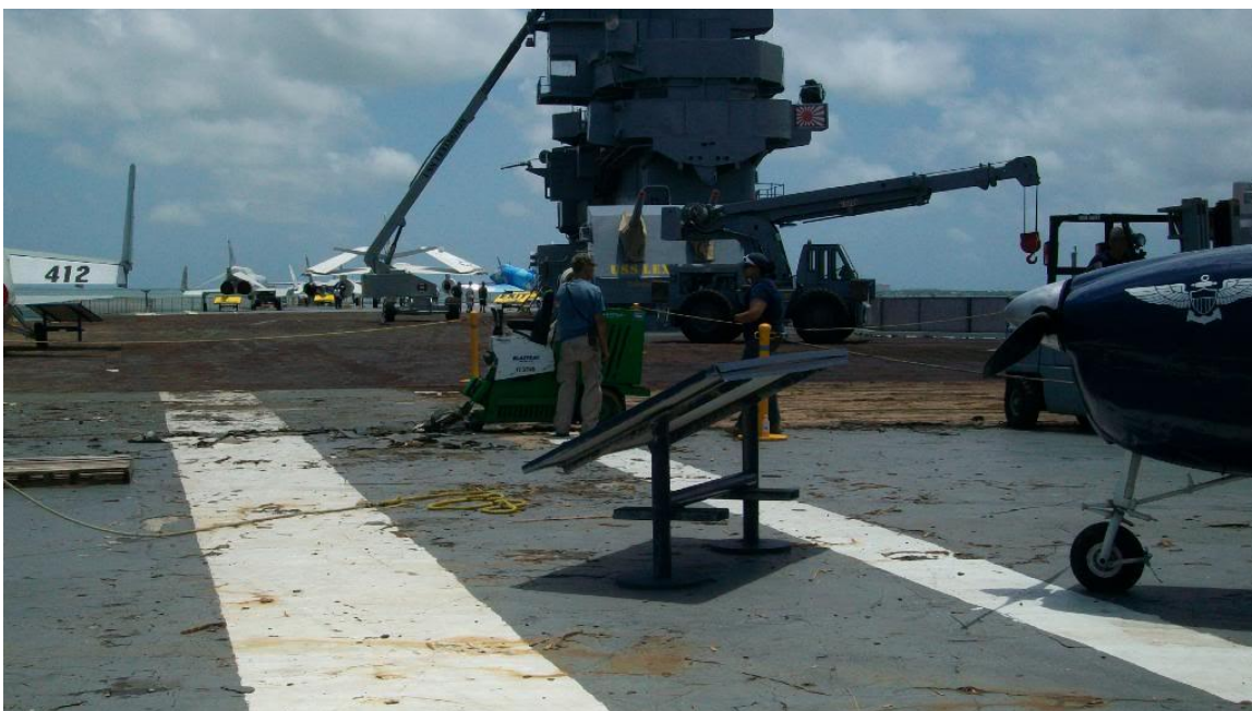
Photograph 85: Museum staff removing the rubber coating from the flight deck.
