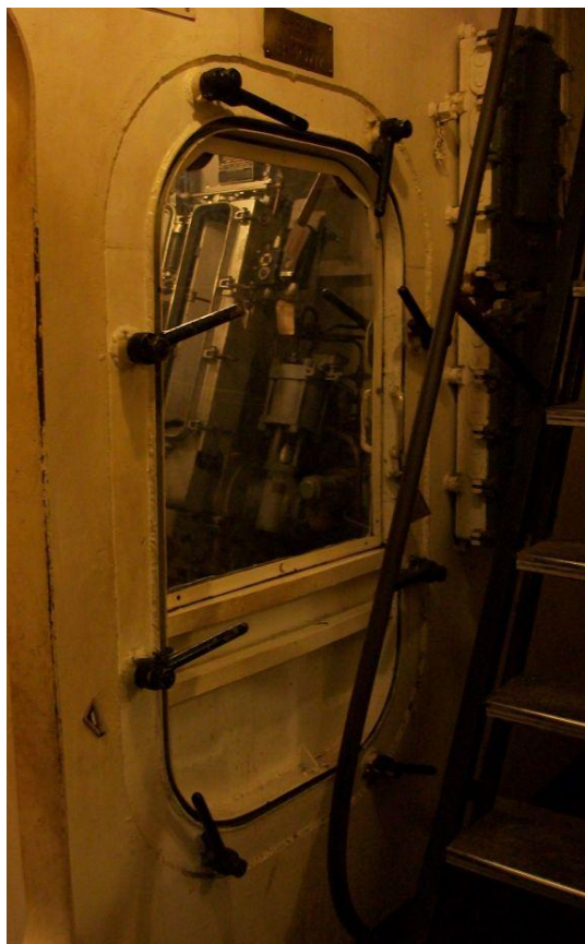
Photograph 23: Lower Handling Room for a starboard 5'' turret, with hatch partially removed for viewing. The addition of ladders along the tour route occasionally poses obstructions.
