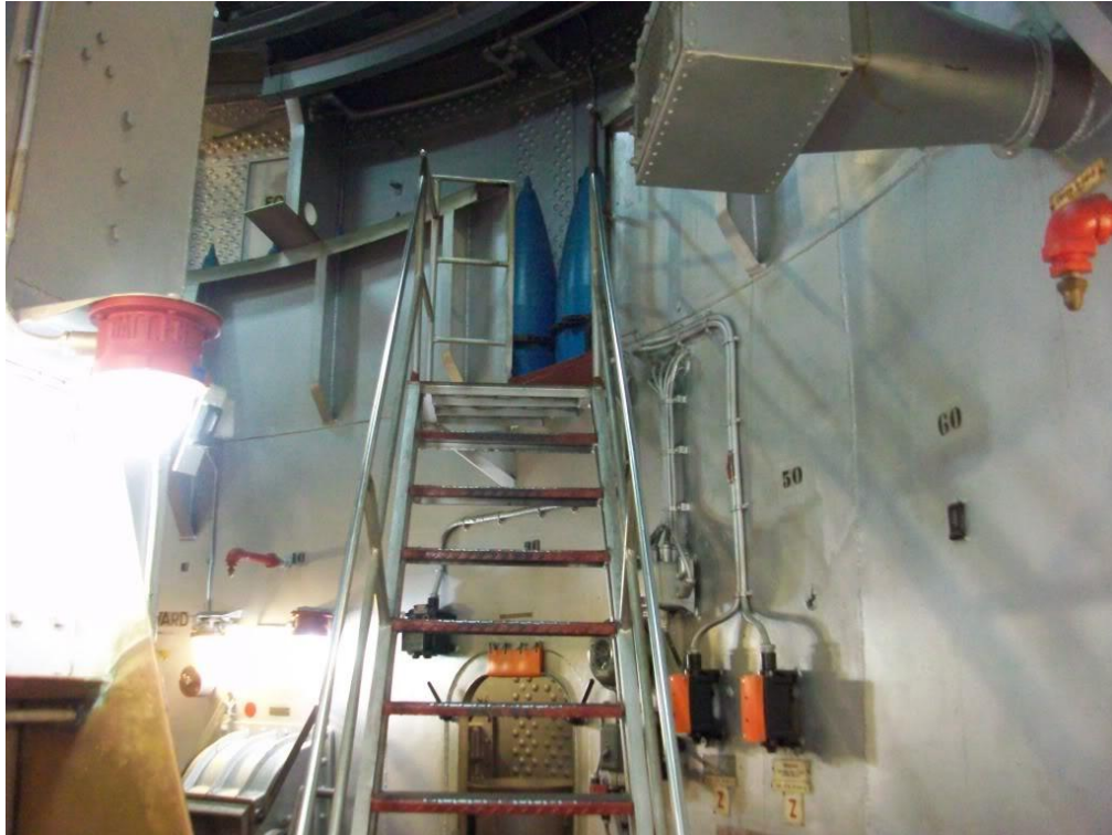
Photograph 17: Reverse view of access ladder.
