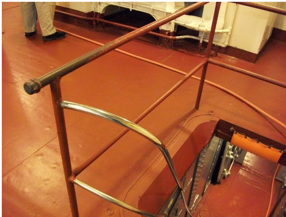
Photograph 24: Detail of railings installed by the museum for visitor safety and access.
