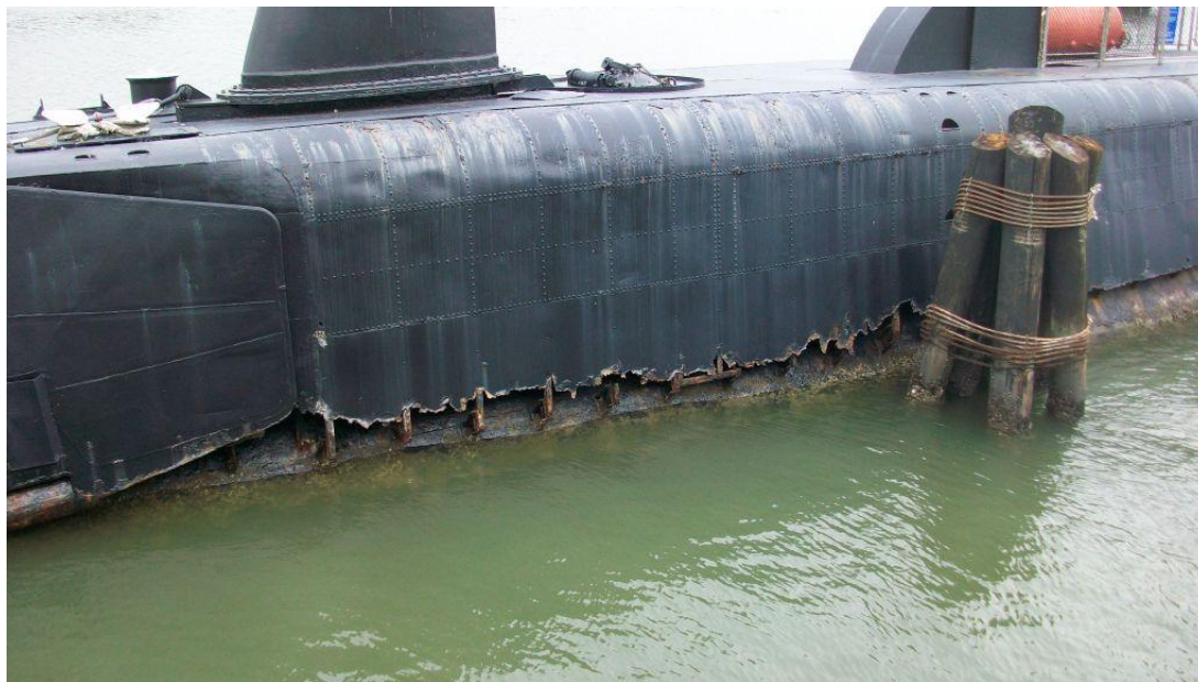
Photograph 55: Corrosion on Clamagore 's hull, September 2011.
