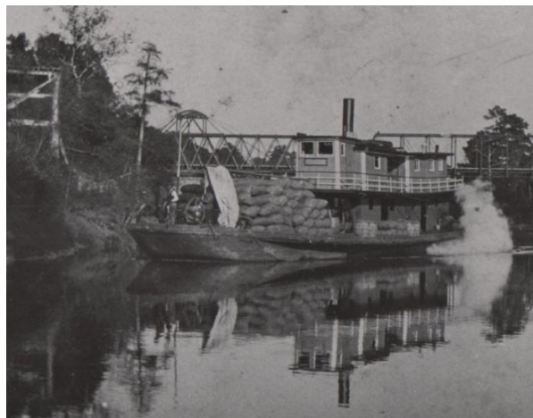
FIGURE 27. Photograph of upriver steamboat Shiloh on the Tar River (Courtesy of Bridgers Collection, Outer Banks History Center).
