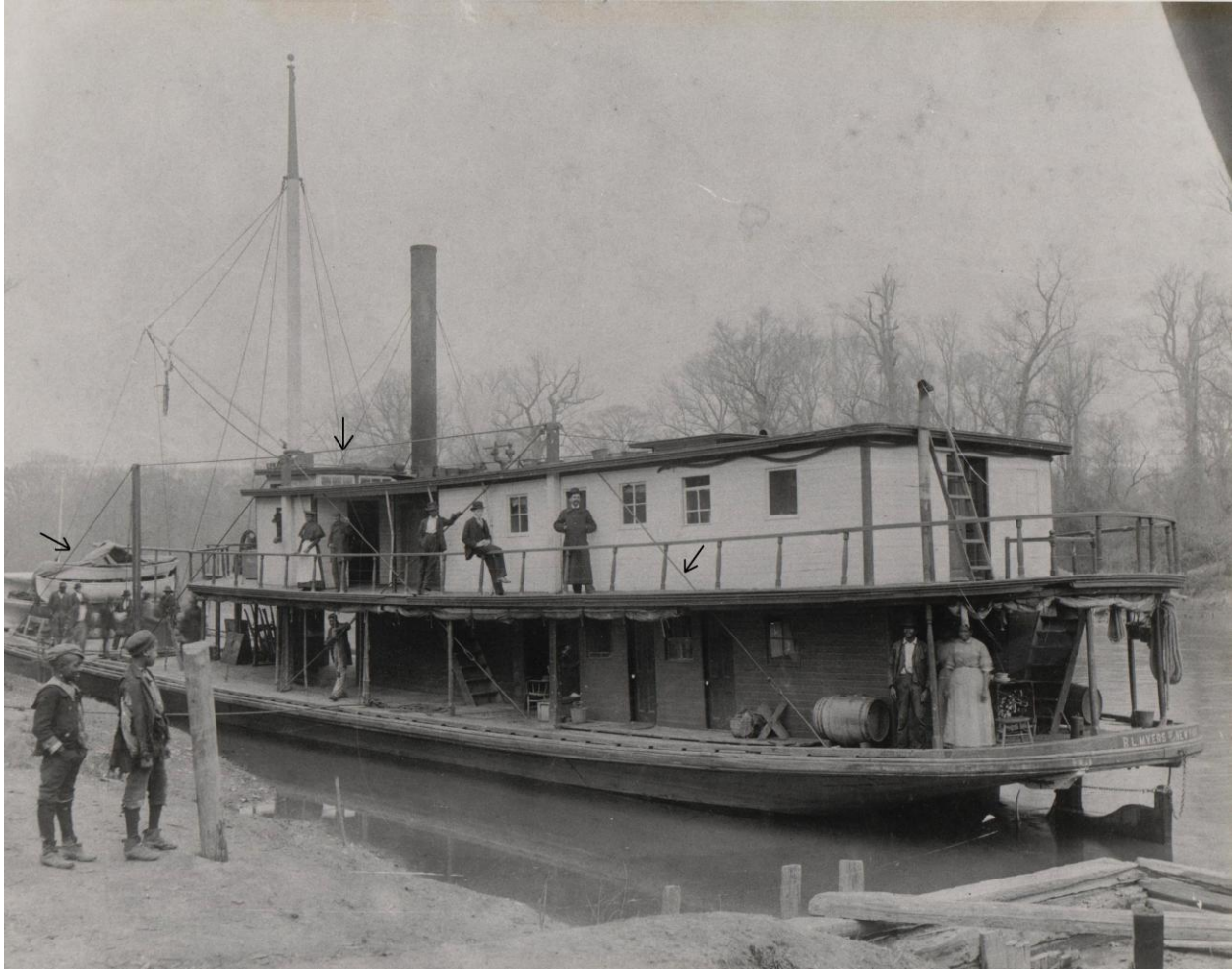
FIGURE 39. Photograph of R. L. Myers (II) at Tar River Landing ca. 1897. Note the hogging chains indicated by arrows (Courtesy of Bridgers Collection, Outer Banks Historical Center).
