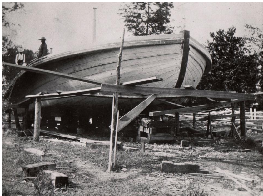
FIGURE 38. Upriver steamboat, believed to be Tarboro (II), under construction as seen from the bow (Courtesy of Bridgers Collection, Outer Banks History Center).
