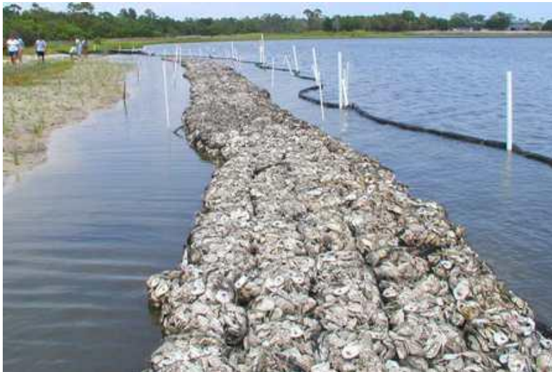
Figure 6. Living shoreline with an oyster sill at Morris Landing in Onslow County, North Carolina.
