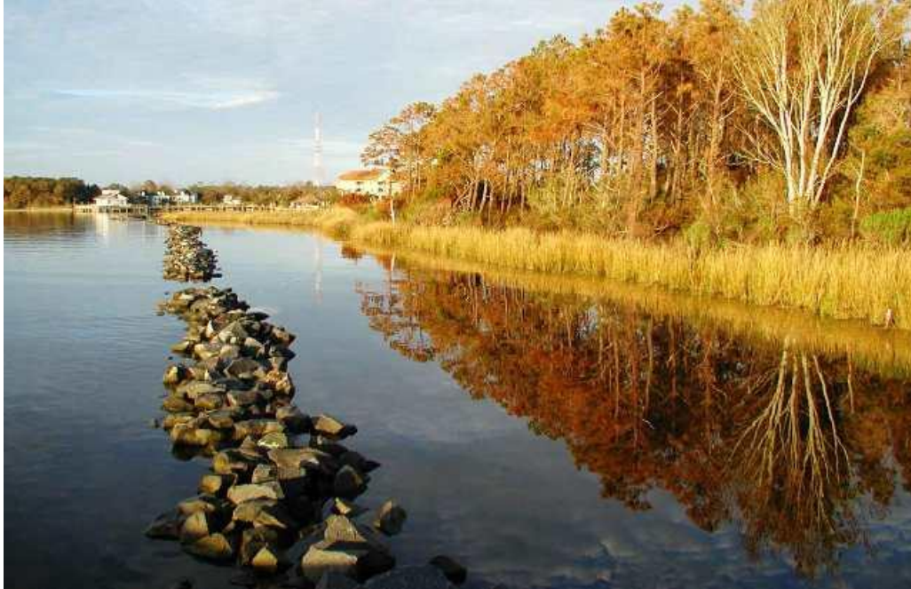
Figure 5. Living shoreline with a rock sill at Roanoke Island Festival Park in Manteo, North Carolina.
