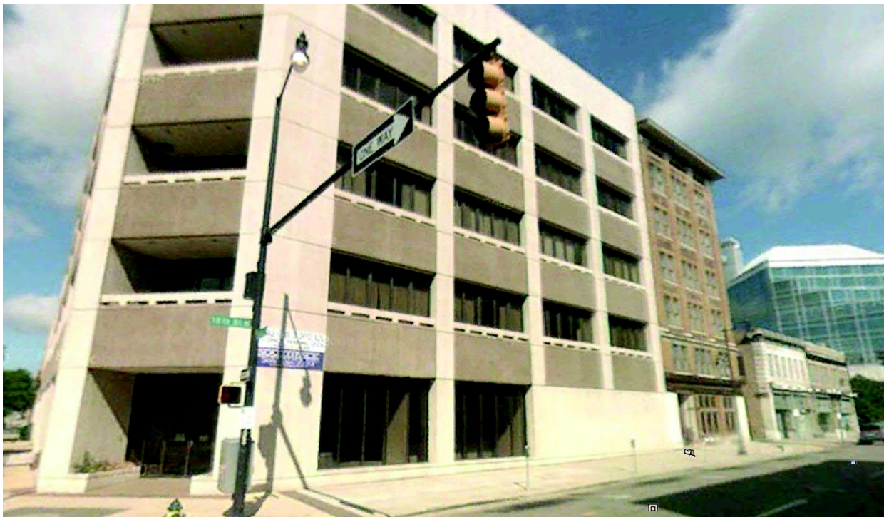
Figure 30 Building now occupying location of Palm Leaf Hotel Birmingham, AL (Google Earth 3D 2013)
