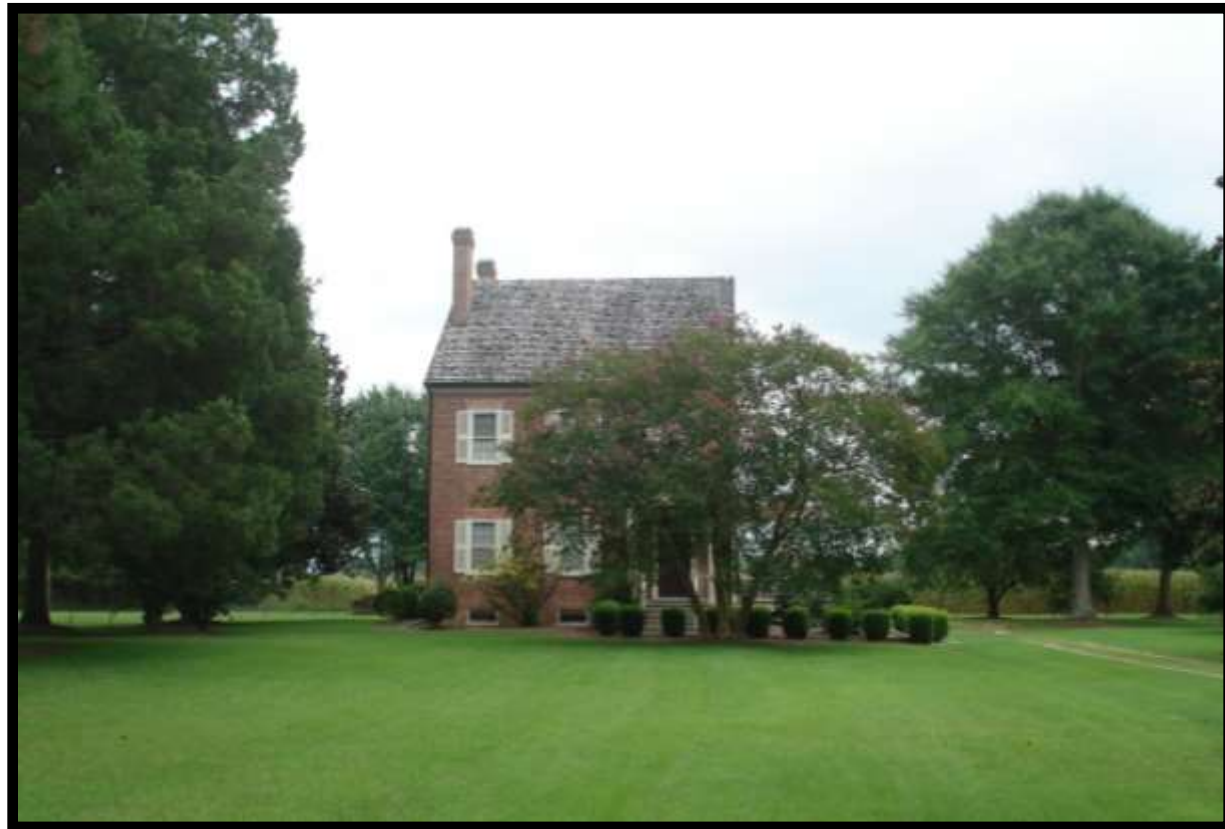
Figure 1-2. Extant Foscue Plantation Main House, Looking East.
