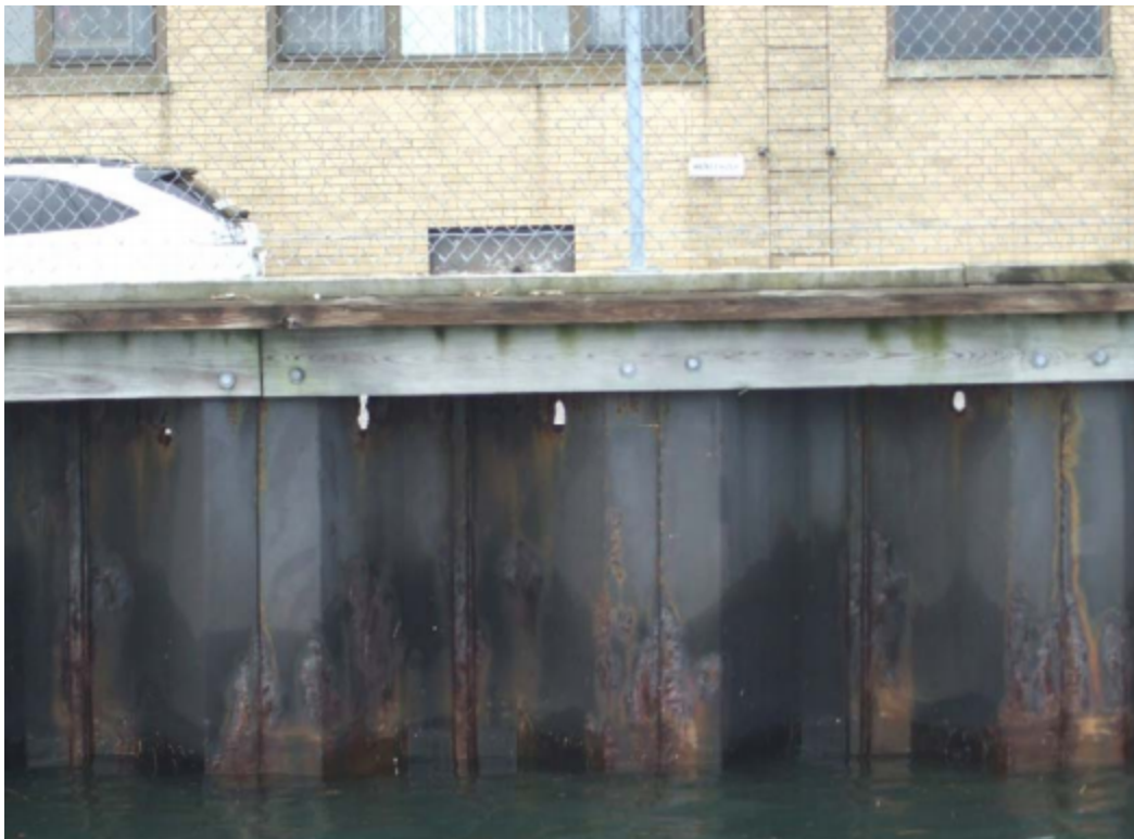
Figure 3.6: Bulkheads of inferior quality. Courtesy of Coastal Planning & Engineering: Bayside Flood Protection Plan 2009
