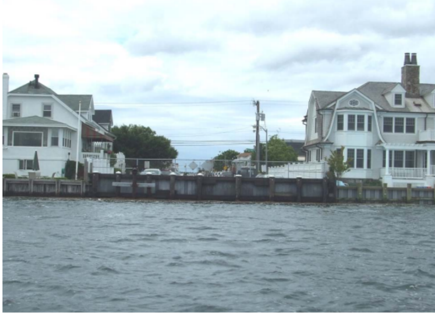
Figure 3.5: Bulkheads in the study area of differing elevations. Courtesy of Coastal Planning & Engineering: Bayside Flood Protection Plan 2009
