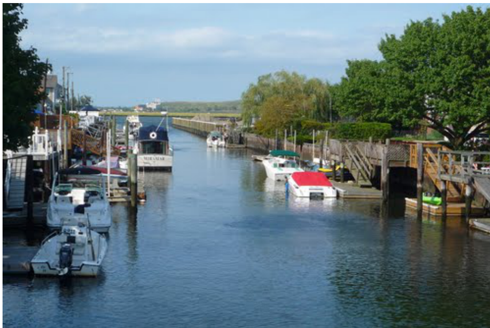
Figure 3.4. Photograph of a canal at ground level
