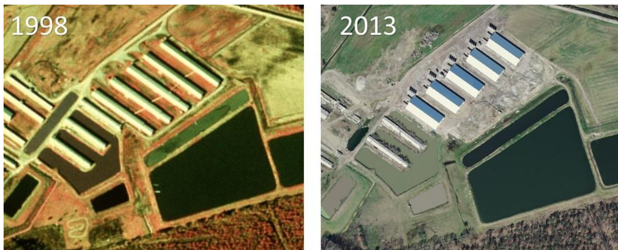
Figure 30: Rebuilt swine housing structures in vulnerable locations after 1998, on swine farm AWS740006.
