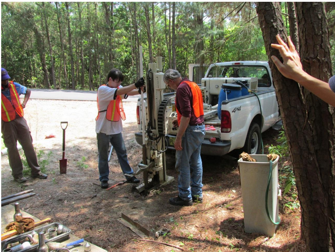
Figure 5: The author (middle) installing a well using the Geoprobe.
