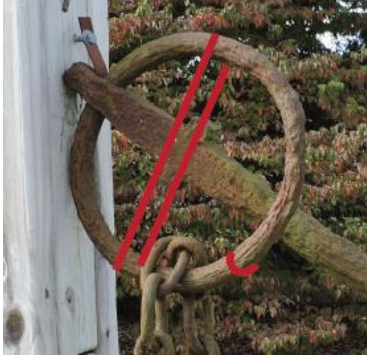
FIGURE 40. BNC002 showing the ring diameter, ring eye diameter, and ring thickness measurements (Marlowe 2016).
