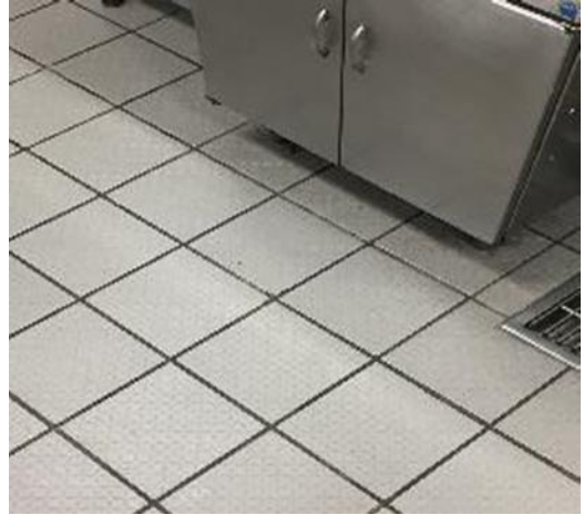
Dining Hall 4 fryer area measured tiles.
