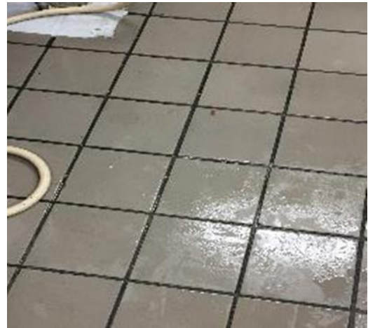
Dining Hall 2 sink area measured tiles.
