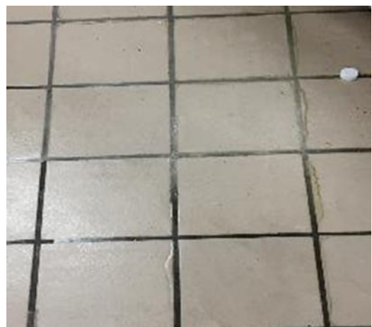
Dining Hall 2 oven area measured tiles.
