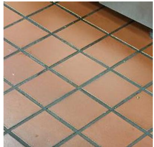
Dining Hall 1 fryer area measured tiles.
