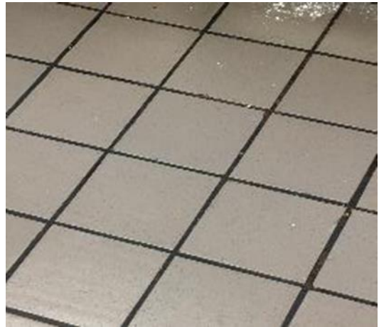
Dining Hall 3 fryer area measured tiles.
