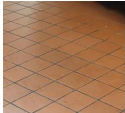
Dining Hall 4 front counter area measured tiles.
