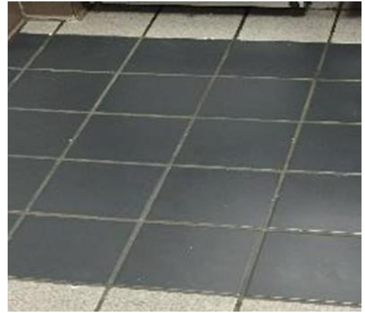
Dining Hall 3 front counter area measured tiles.
