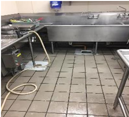
Dining Hall 2 sink.
