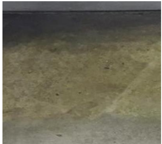
Dining Hall 2 front counter area measured floor.
