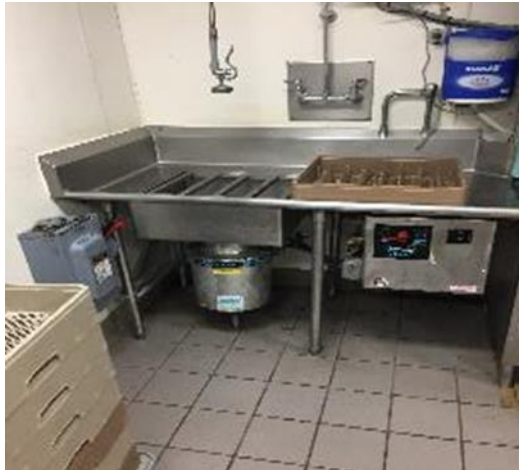
Dining Hall 4 sink.
