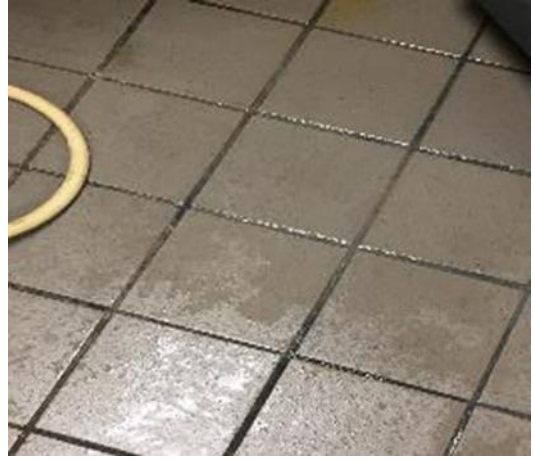
Dining Hall 3 sink area measured tiles.
