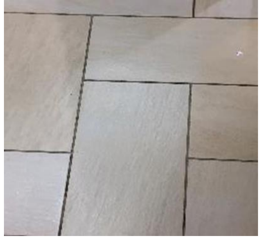
Dining Hall 1 front counter area measured tiles.
