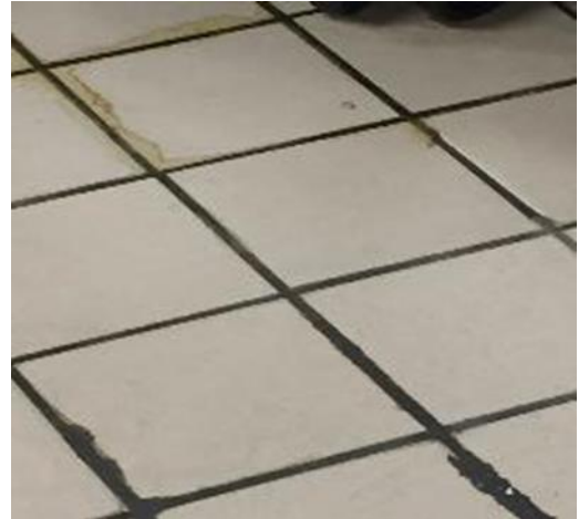
Dining Hall 2 fryer measured tiles.
