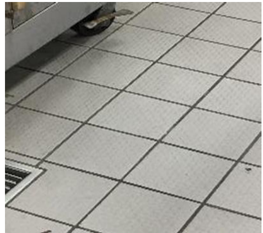
Dining Hall 4 oven measured tiles.
