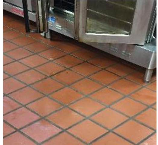
Dining Hall 1 oven area measured tiles.
