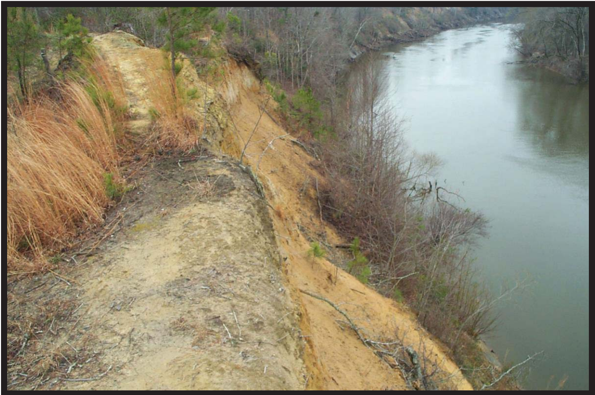
Figure 22: Erosion on the Interior of the Fort.
