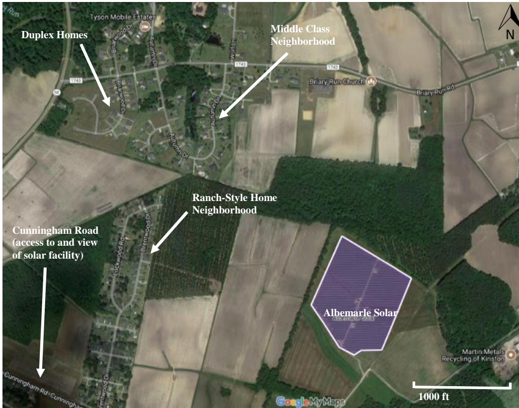
Figure 8: Albemarle Solar Center study site
