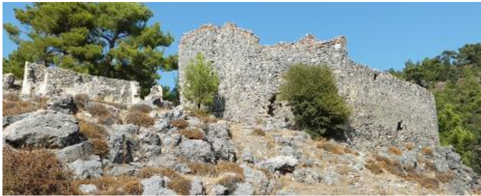
FIGURE 5.22 Ruins of structure facing due north (Photo by Eray Salioglu 2017)
