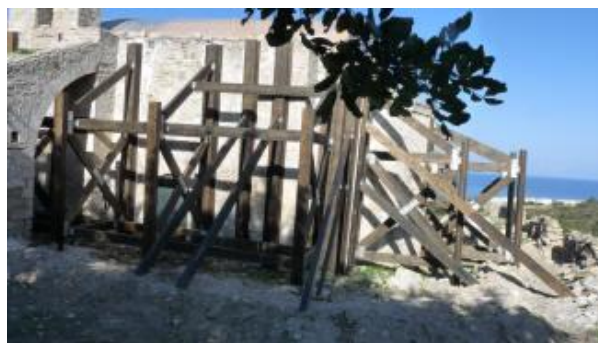
FIGURE 5.62 Melandryna Monastery repairs (Watson-Northcyprus 2018)
