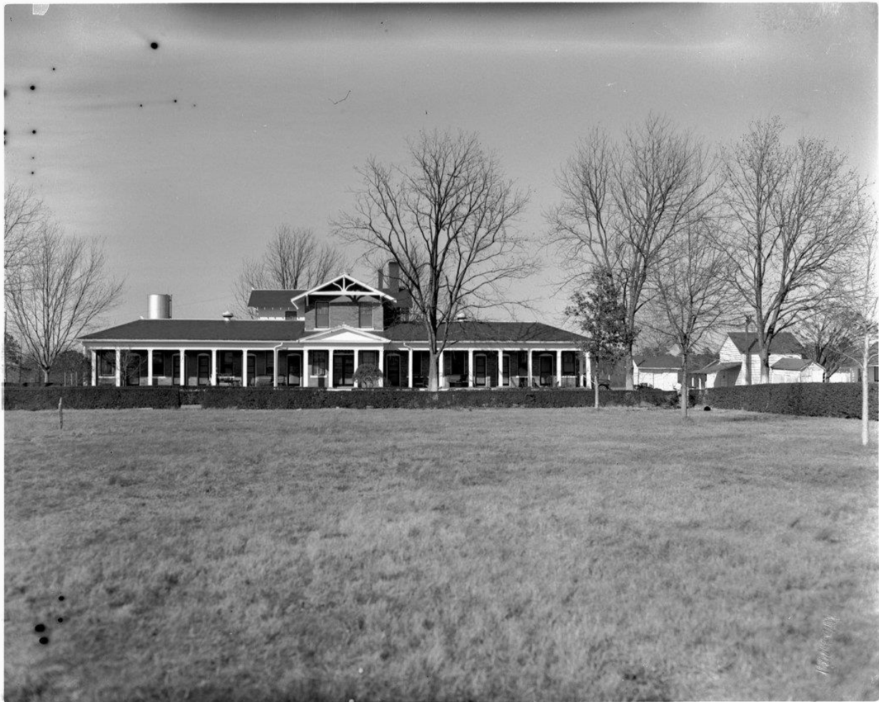
Figure 27: Picture of the southern face of the main building from the second Pitt County Poor Farm with outbuildings in the background (Rhodes 2016).
