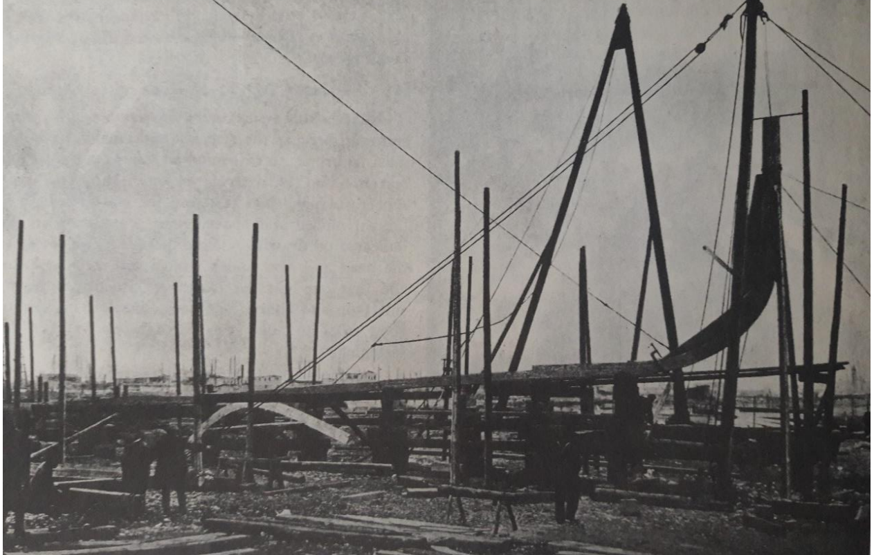
Figure 4. Keel set up (Desmond 1919:48).
