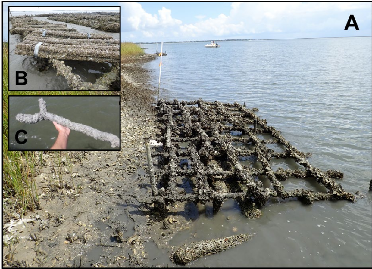
Figure 1.2: Schematic of a novel OC reef and its components. A) Each OC reef, such as this example on the ramp shoreline, was designed as a raised latticework composed of B) long, thin rods supported by C) thick, Y-shaped supports, which are sunk into the marsh sediment to the point of refusal. Photo C courtesy of N. Lindquist.
