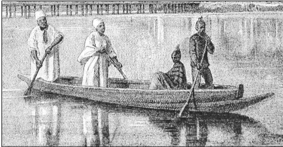
Illustration 3.2.10: Bridge over the Senegal at St. Louis with boat in the foreground 1879-1880, cropped, from (Lenz 1886:335) May have been drawn from firsthand observations.
