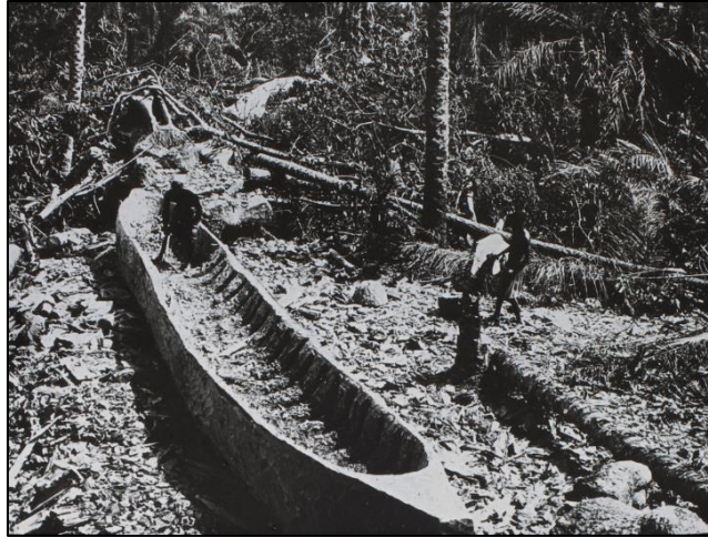
Photograph 4.9.6: Carving the inside of a logboat, Ziguinchor, Casamance From (Tastevin 1900)
