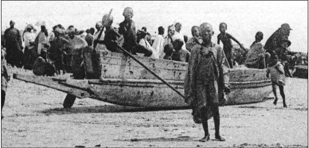
Photograph 4.11.2: Boat with extended cutwater revealing scarfed extension Senegal River Coast Cropped, from (Anonymous Unknown)
