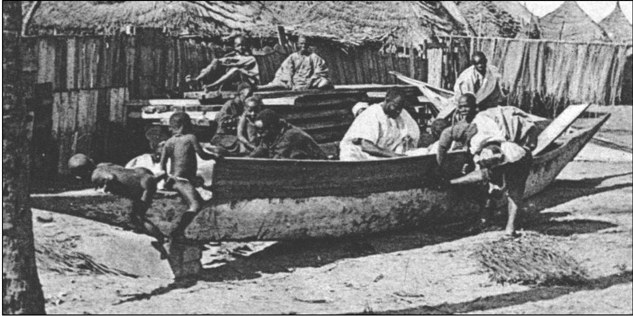
Photograph 4.10.1: Boat under construction on the Cape Verde Peninsula Cropped, from (Anonymous Unknown) A pile of fiber could be seen next to the boat likely used for lashing or caulking. Boat appeared to be supported on one end by logs. Multiple workers work on the boat while observers watch and children play
