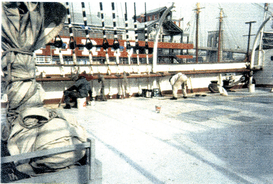
Fig. 14. Workers on deck
