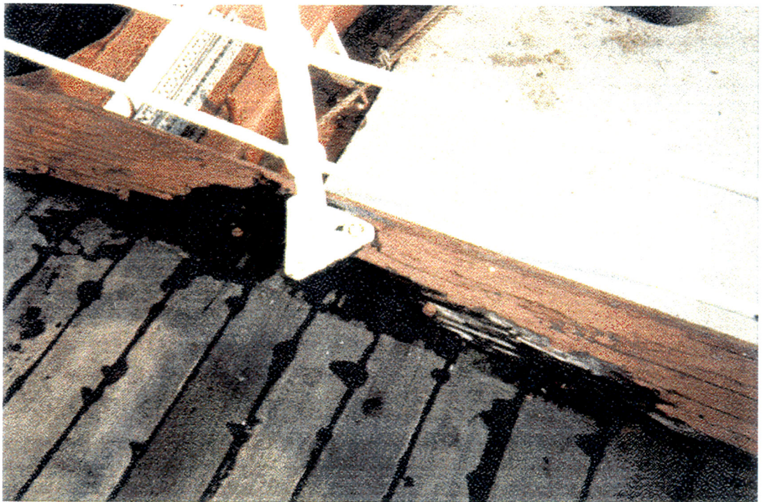
Fig. 13. Damaged wooden railing
