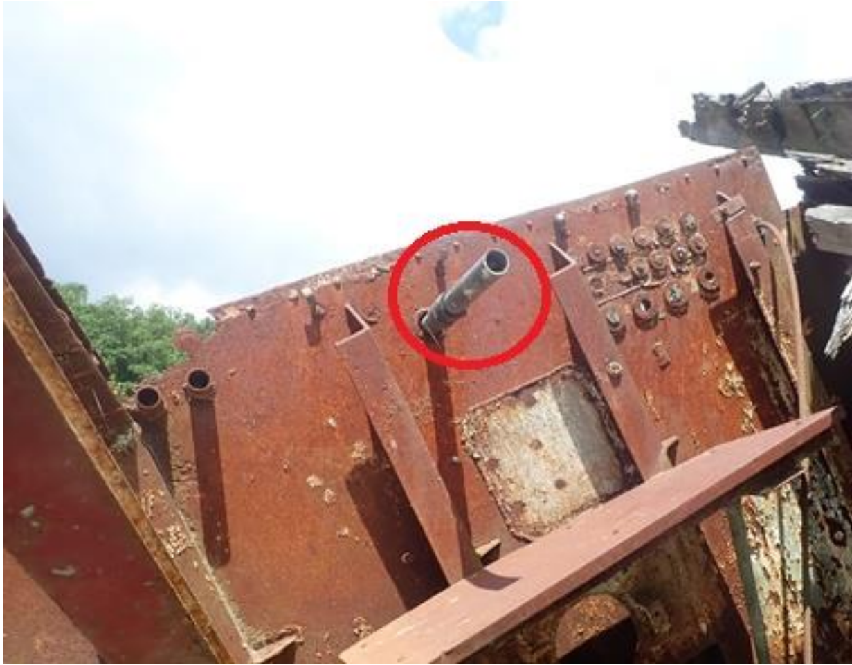
FIGURE 6.12 PVC pipe (circled in red) for electrical wire going through Bulkhead 6 of the Sea Scout Wreck (Facing northeast) (Photo Credit: Nathan Richards, 2021).
