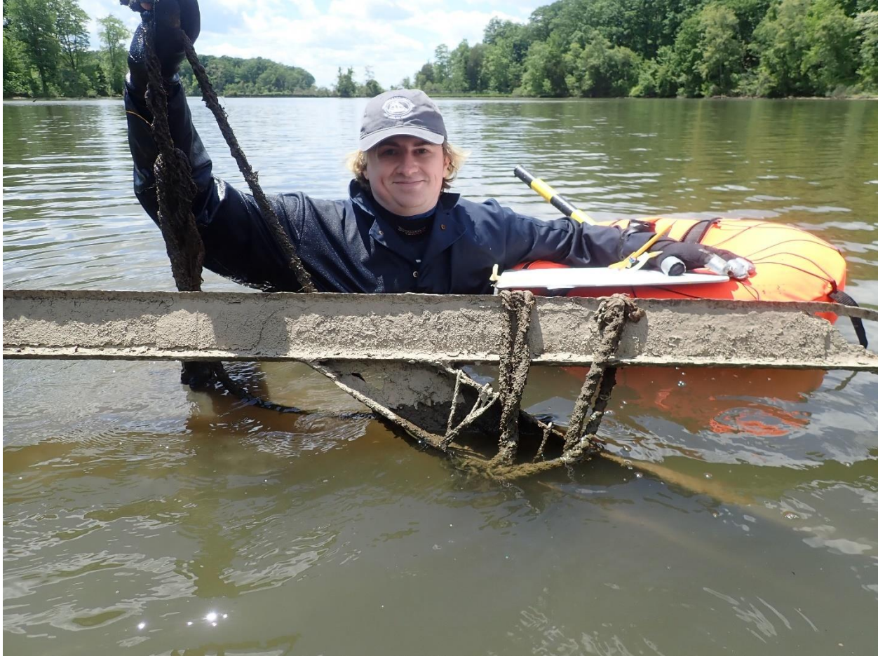
FIGURE 6.29 Taylor Picard holding up a length of broken rope attached to starboard I-beam between Bulkheads 5 and 6; note break in the I-beam on the right (Photo Credit: Nathan Richards, 2021).
