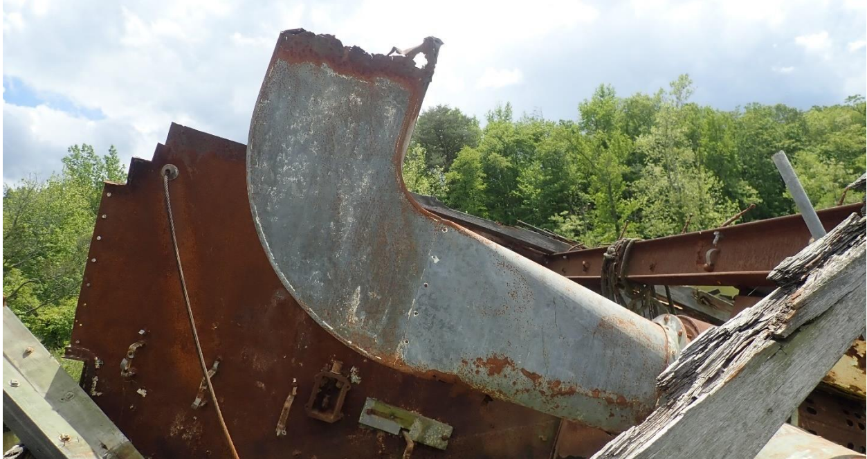
FIGURE 6.10 The ventilation shaft in the engine room of the Sea Scout Wreck. This appears to have originally lined up with the mushroom vent that would have been removed when the pilot house was extended (Photo Credit: Nathan Richards, 2021).
