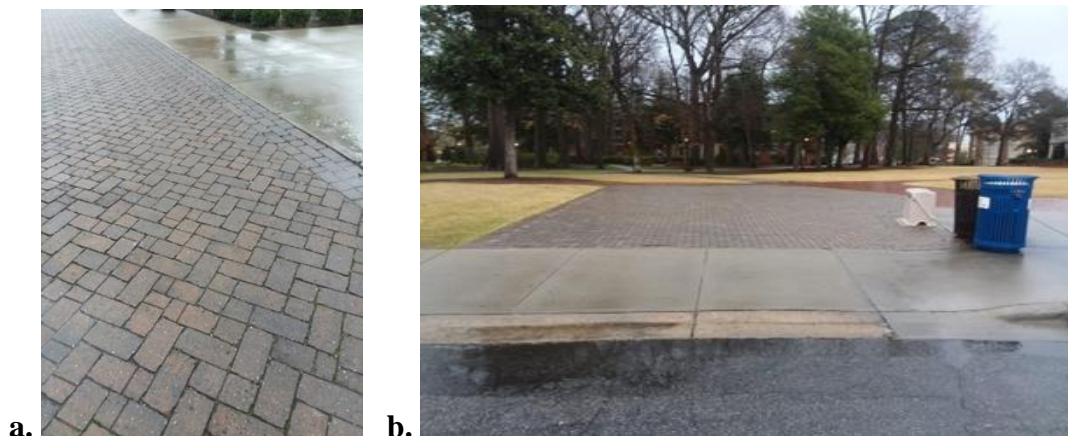
Figure 23. PICP sites show no runoff generation during rainfall events; (a) Student Plaza Drive on February 6, 2020 and (b) Band Shell Plaza on March 3, 2020.
