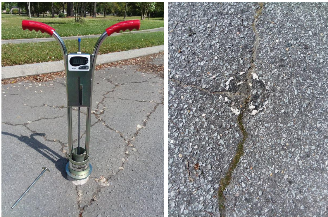
Figure 7. Typical setup of double-ring infiltrometer at asphalt sites.
