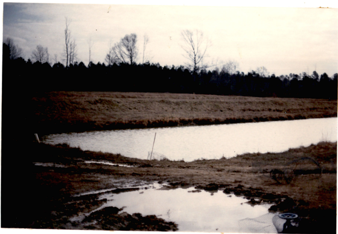
FIGURE 16. Production ponds at Buck Trail Aqua Farms. Note the alternating excavated and diked pond construction.
