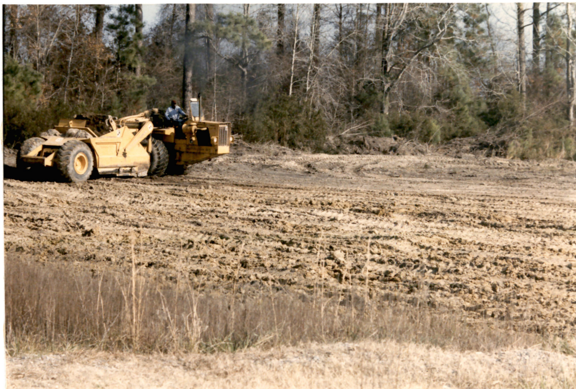
FIGURE 5. Diked ponds under construction at the Pamlico Estaurine Laboratory, Aurora, NC. The topsoil is removed and the ground scooped out to a depth of one or two feet. The spoil is used to construct the dikes.
