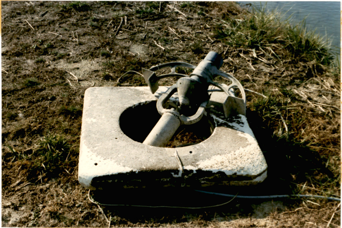
FIGURE 9 A. Floating electric aerator.
