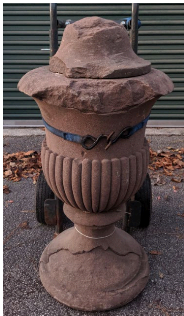
Figure 4.03: The Rhem Vault urn after it fell from the roof. Photo provided by the Rhem descendants.
