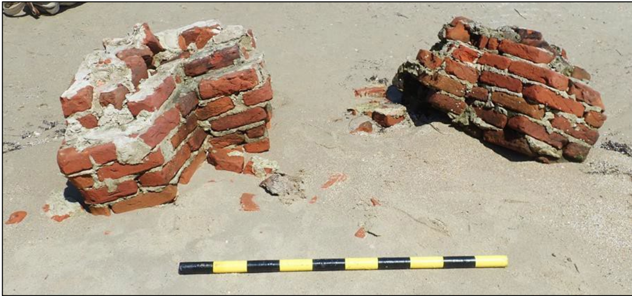
FIGURE 5.5: P6180028, 06/17/2021, scale bar is one meter. photo taken by Jill Schuler of a brick structure (Schuler 2021).
