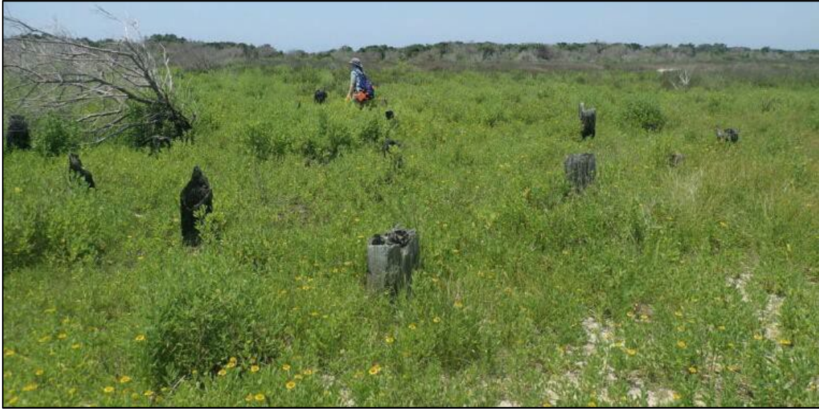
FIGURE 4.6: Photo P6200012, taken by John Detlie, depicting the structure remains of a house that was likely burned by locals when the NPS took over (Detlie 2021).
