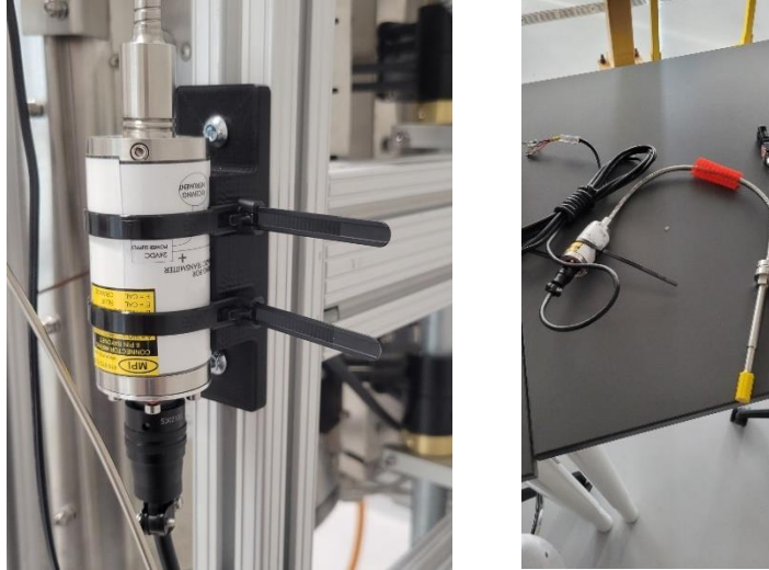
Figure 145: 3D printed bracket with mounted pressure sensor support electronics enclosure on the 100mL/min desalination system.
