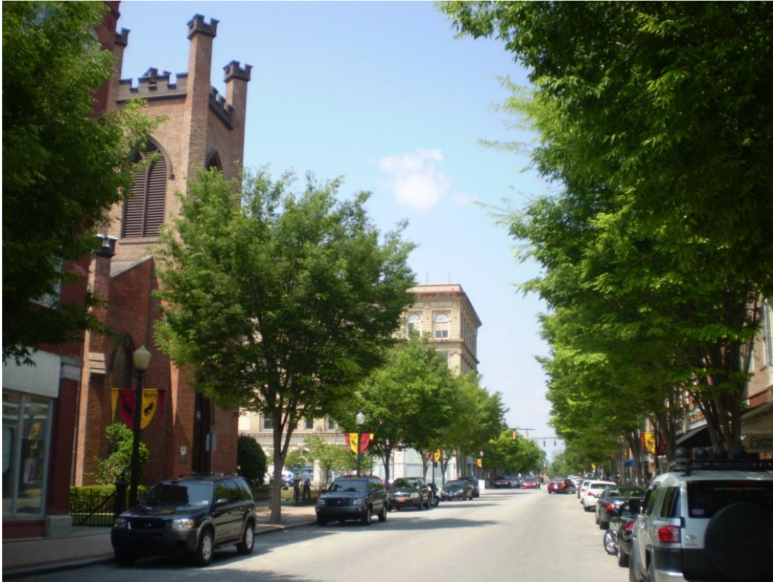
Figure 8: Looking north down Middle Street. Although every building pictured here is brick, varying colors and shades provide variety. Note the difference in brick caused by the sun on the 1 st Baptist Church at the left. The tan-bricked Elks building can be seen in the background.
