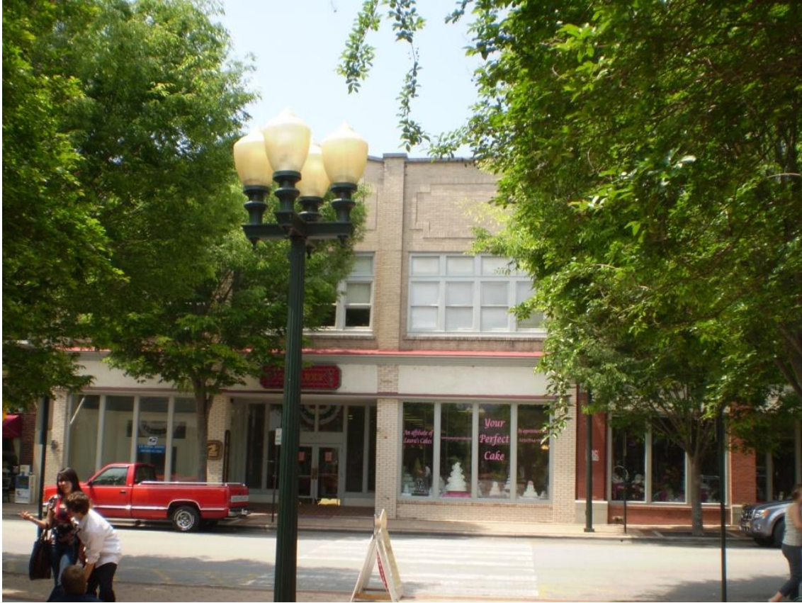
Figure 5: The O. Marks Building is a textbook example of adaptive reuse. Once a building for a Belk department store, it was bought by a local partnership when Swiss Bear learned it was being considered by investors for an adult entertainment center.
