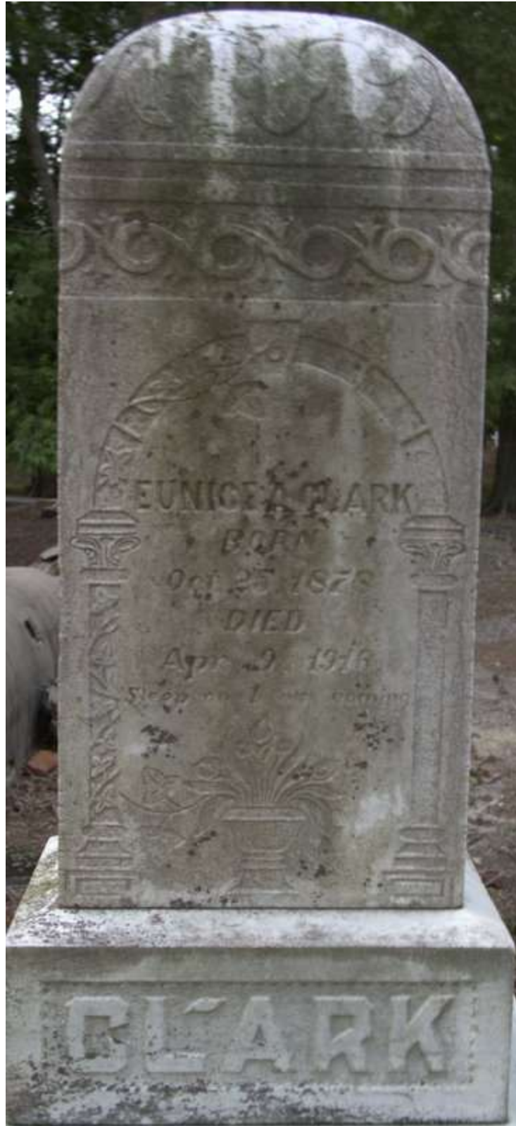
Figure A.3. Marble stone showing staining which hinders readability.
