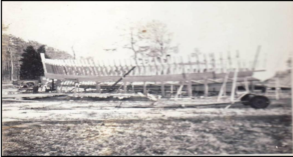
FIGURE 145. Shell-first construction practiced by boatwrights of Wright's Creek, this shell constructed by Major Wilson Foster Ca. 1964 (Carl Wilson Foster Collection, Belhaven, NC).
