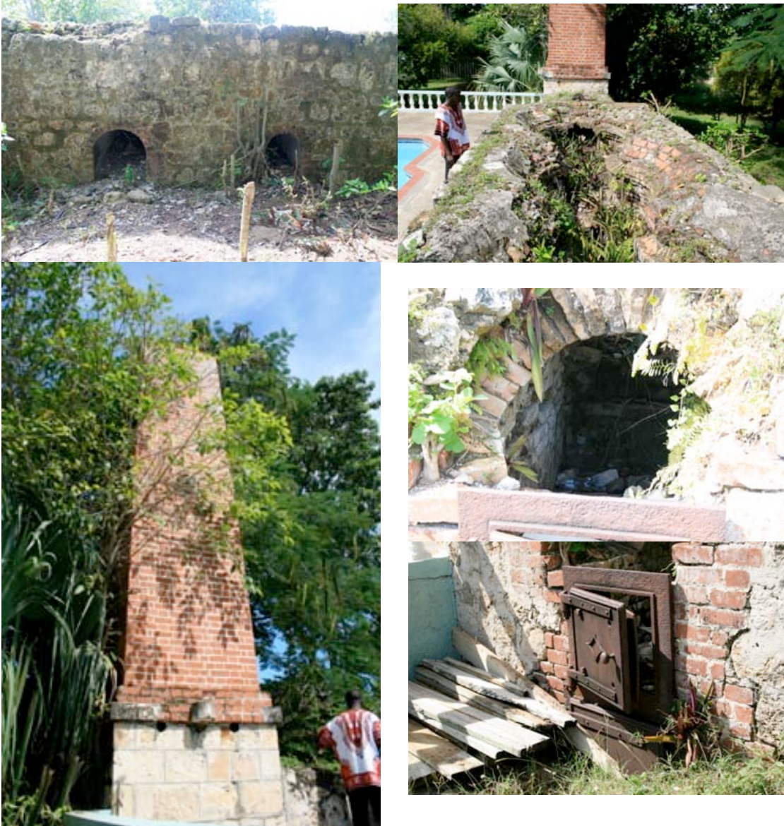
FIGURES 84 top left , 85 top right , 86 middle right , 87 bottom right , and 88 bottom left . The Kiln's: eastern stoke holes, burning pits, southern flue, metal door, and red brick chimney respectively. Notice the modern pool just adjacent to the west side of the kiln, visible in Figure 85. (Photos by Peter Campbell, November 6, 2009.)
