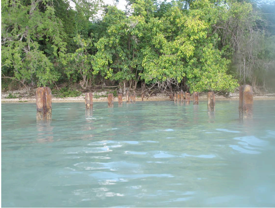
FIGURE 53. Interior of the Southern Group of I-beam Pilings. Shot from their western extent facing east. Photo by author, October 25, 2009.)
