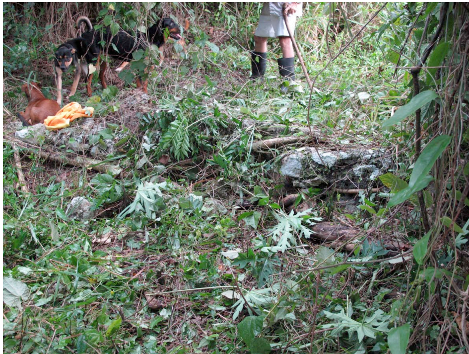
FIGURE 44. Interior of the eastern wall of the Oristano Structure. (Photo by author, October 30, 2009.)
