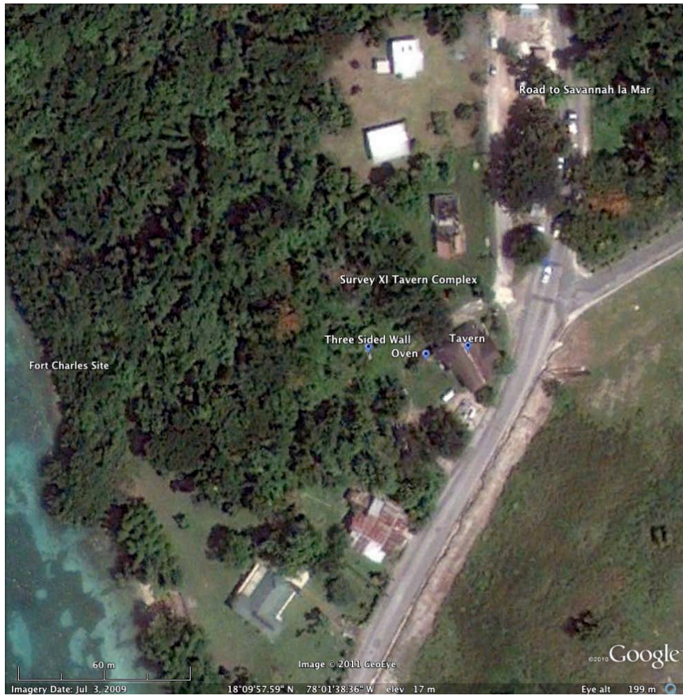
FIGURE 60. Survey XI Results. Survey XI covered three buildings, the Bluefields Tavern , an adjoining Oven , and a three-sided wall nearby. Note the tavern's proximity to the road to Savannah-la-Mar . (Map by author, 2009.)
