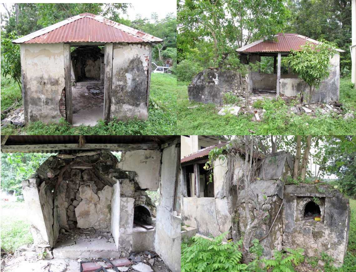
FIGURES 65 top left , 66 top right , 67 bottom right , and 68 bottom left . Views of the Oven Building's north, east, and west sides, and an interior view of the oven from the south respectively. Notice the brick oven attached to the southernmost wall of the structure. In Figure 65 it appears to have two oven openings, a larger one on the left, and a smaller one on the right. (Photos by author, October 26, 2009.)
