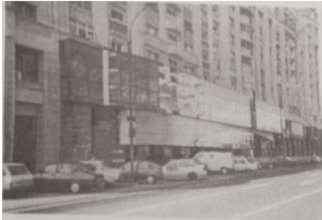
The offices of "The Romanian Commercial Bank" on "Calea Victoriei"-The modified ground floor of a former block built during the last part of Ceausescu's regime
