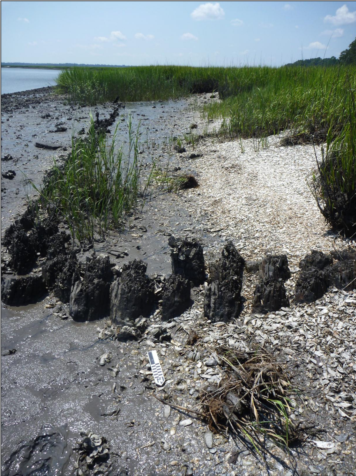
FIGURE 5.7: Closed double piling reinforcement turning into the marsh at Lamotte's Wharf (Photo by Joseph Roberts).
