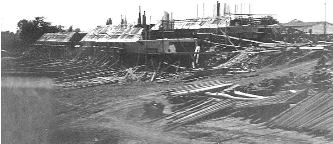
FIGURE IV.3. Four “City-class” Union ironclad gunboats being constructed at St. Louis, Missouri prior to October 1861. They will be launched sideways into the river. The construction process for these ironclads was similar to that used for regular steamboats. (Online Library of Selected Images, Naval Historical Center, Department of the Navy, Washington, DC, 2012)
