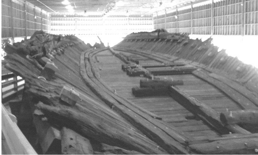
FIGURE VI.43. Until June 2012 the remains of Neuse lay under a roofed enclosure in Kinston, North Carolina, not far from the Neuse River. The remains of the engine, boiler, and propeller shaft mounting timbers can be seen in this view from the stern. Neuse has now been moved to an indoor climate-controlled facility. (Photo by author 2010)
