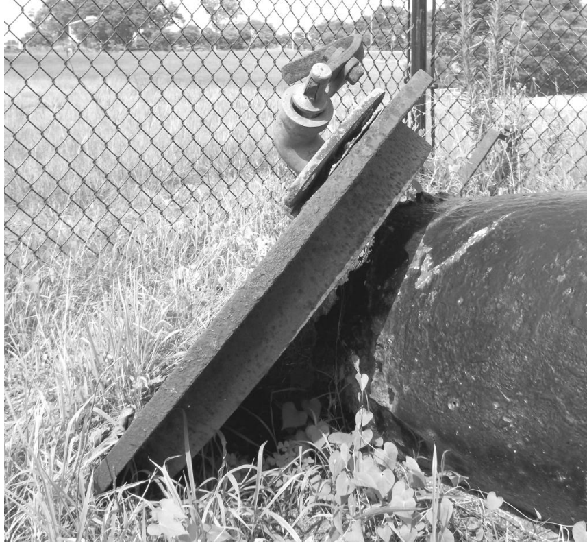
FIGURE VI.63. Side view of the cylinder head, showing thickness of solid iron construction. (Photo by author 2011)
