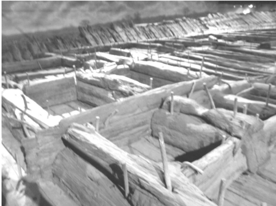
FIGURE VI.57. Large timbers for supporting the engine mounts of Jackson as preserved today. They are approximately 12 inches square. The boiler bed mountings were farther forward, but those timbers were not preserved. (Photo by author 2011)
