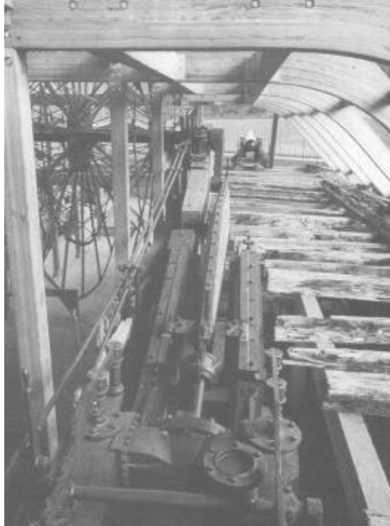
FIGURE VI.47. A view looking aft along the reconstructed Cairo 's port side gundeck, showing the port engine and pitman arm angling up through the deck to connect with the center paddlewheel. The internal arrangement of Missouri would have been similar. (Sheppard 1990)
