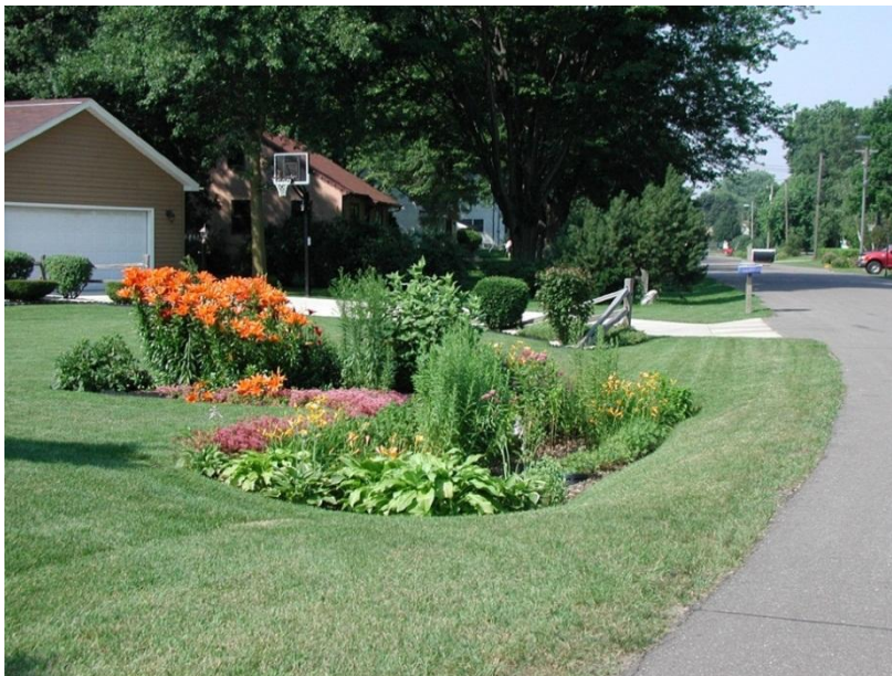
Figure 25: Bioretention garden built in a residential property (from AWPA, 2008)
