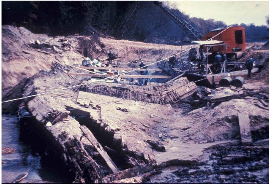
Figure 3.0 CSS Neuse Excavation 22
