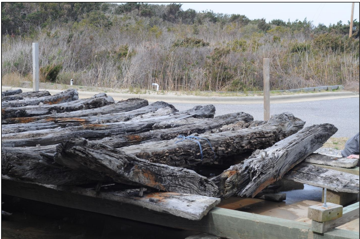
FIGURE 152. The aft most frame has completely collapsed and continues to disintegrate. (Photo by Author 2012)
