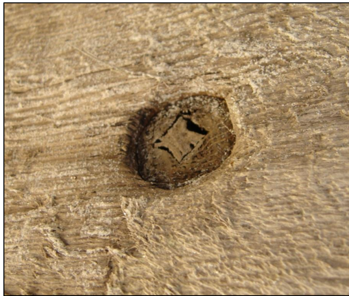
FIGURE 148. Another square-wedged treenail. (Photo by Brad Rodgers, 2010)
