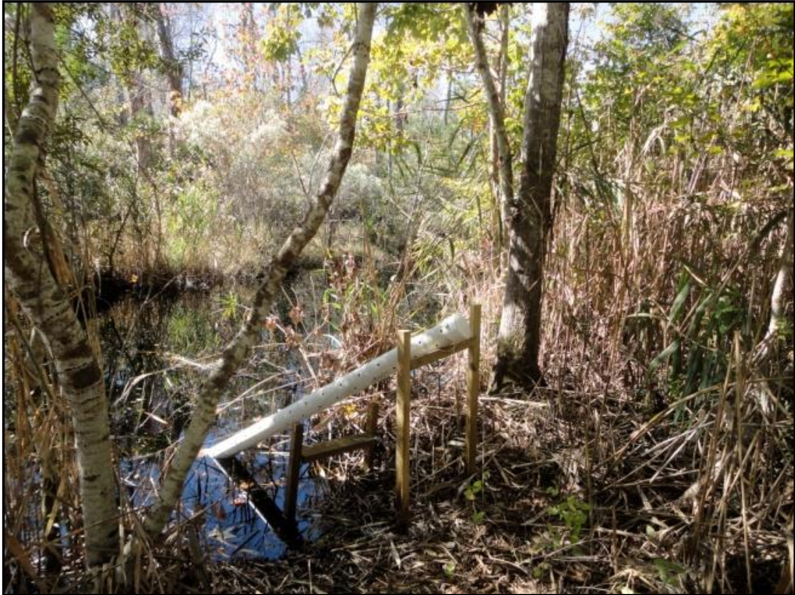
Figure 2-5: Example of a stilling well (SW6) installed in the canal on Buckridge Road.
