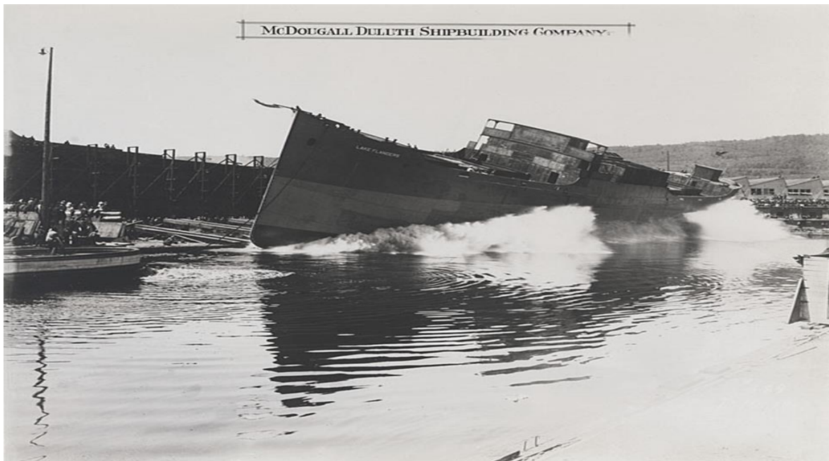
FIGURE 3.5. McDougall-Duluth Shipbuilding Company launching Lake Flanders , Nov. 1919 (University of Wisconsin Digital Collections, Great Lakes Maritime History Project, October 2013).
