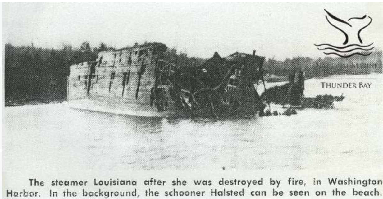
FIGURE 4.1. Total loss Louisiana in foreground, stranded vessel Halstead in background (Swayze 2014).
