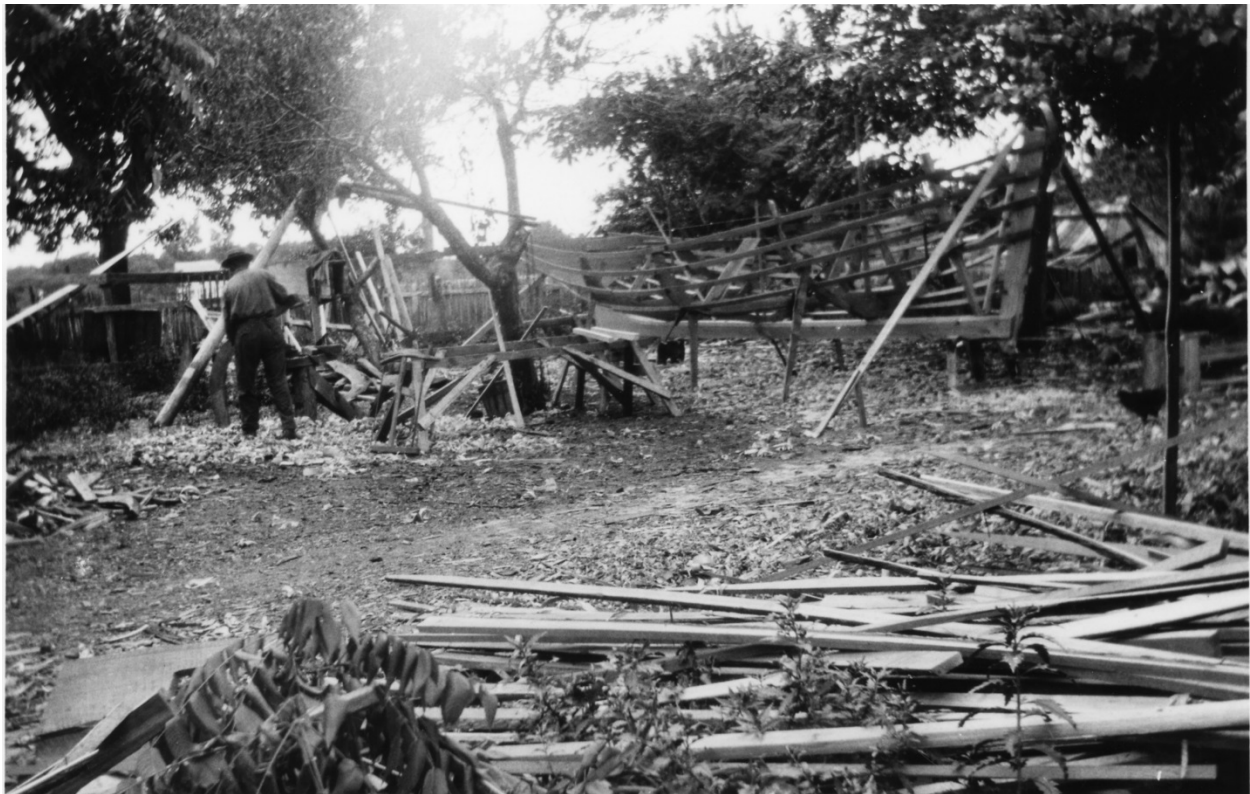
FIGURE 35. Vessel set up for construction with battens and stretchers (Image courtesy of Earl Willis Jr.).
