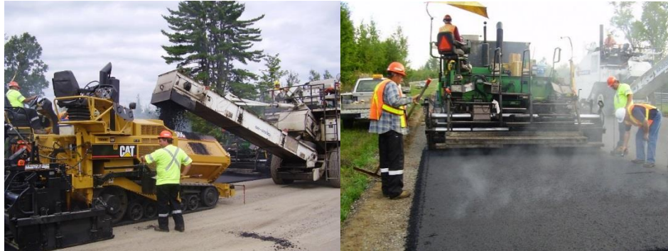
Figure 8: HL8 binder course paving. Figure 9: Echelon paving and material transfer vehicle were employed for surface paving and temperatures were checked constantly.
