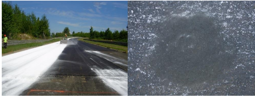
Figure 10: Hydrated lime is applied and rolled. Figure 11: tire mark generated by heavy loaded truck to check the stiffness of HMA surface after approximate one week of paving.
