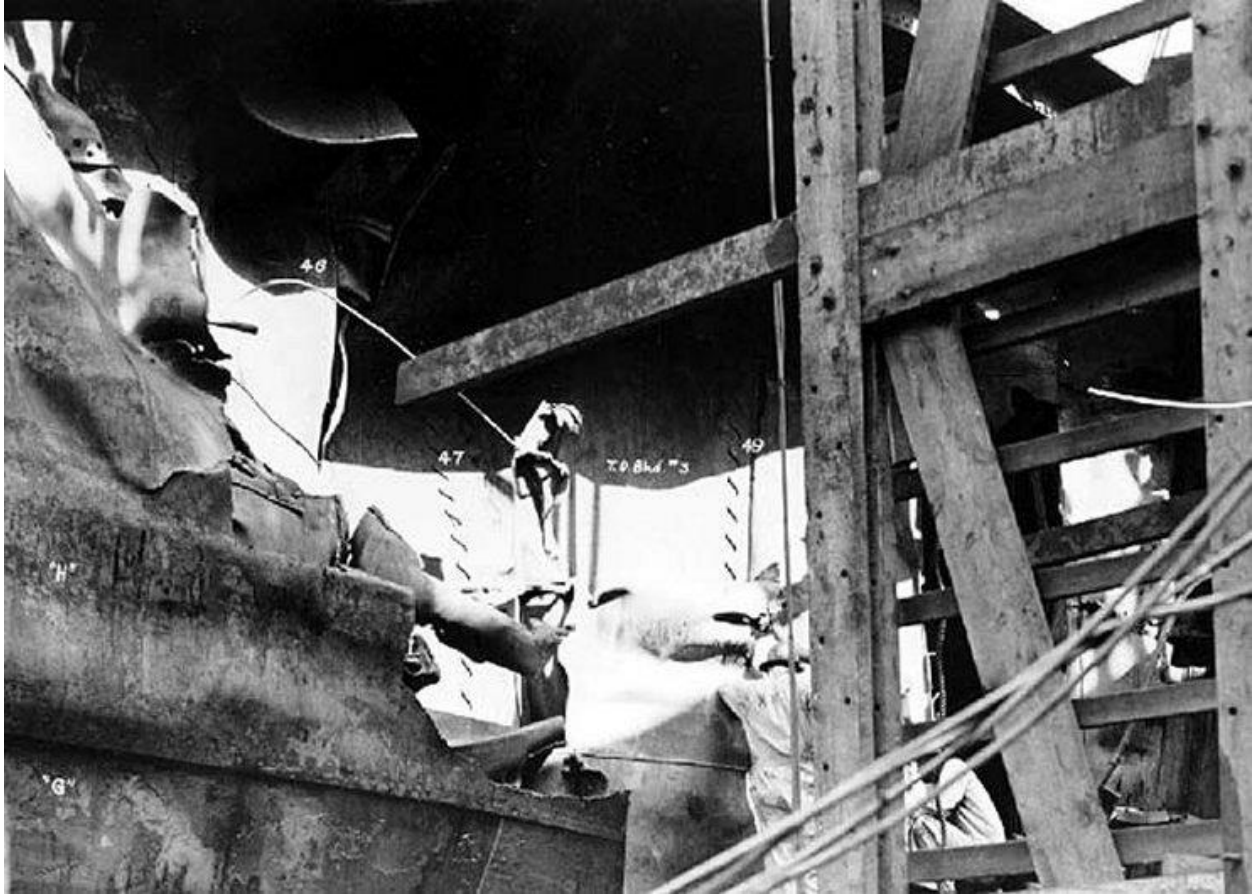
FIGURE 13. Torpedo damage to USS North Carolina (U.S. Navy 1942)
