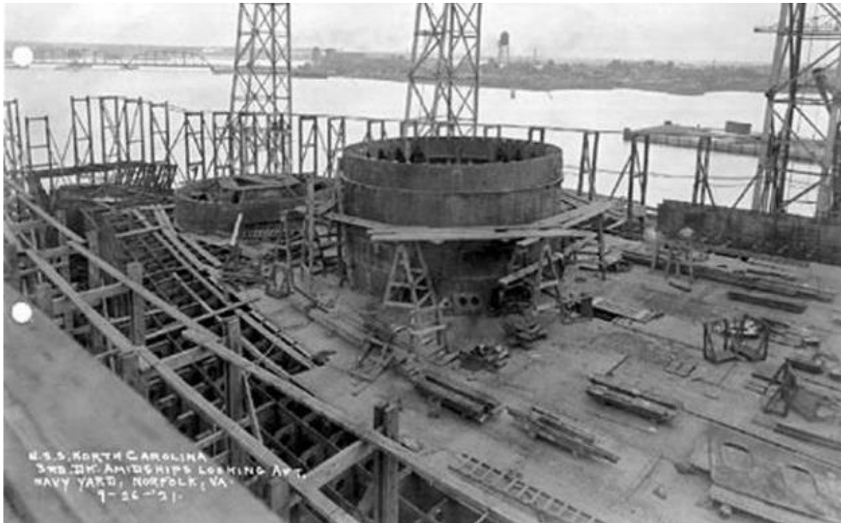
FIGURE 6. USS North Carolina (BB-52), under construction (National Archives 1921)
