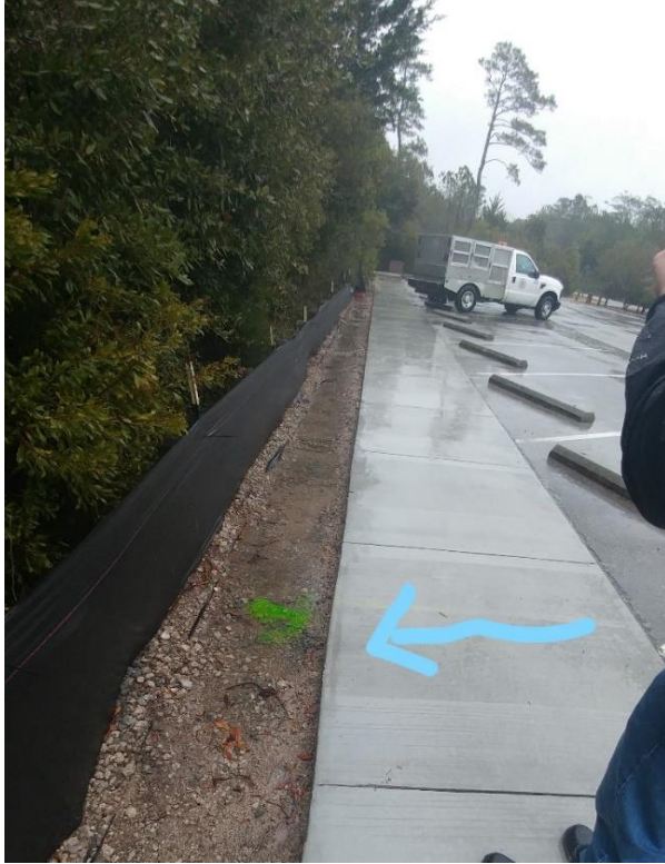
Figure 9: New sidewalk at the boat ramp that was graded to allow runoff to enter the woods.
