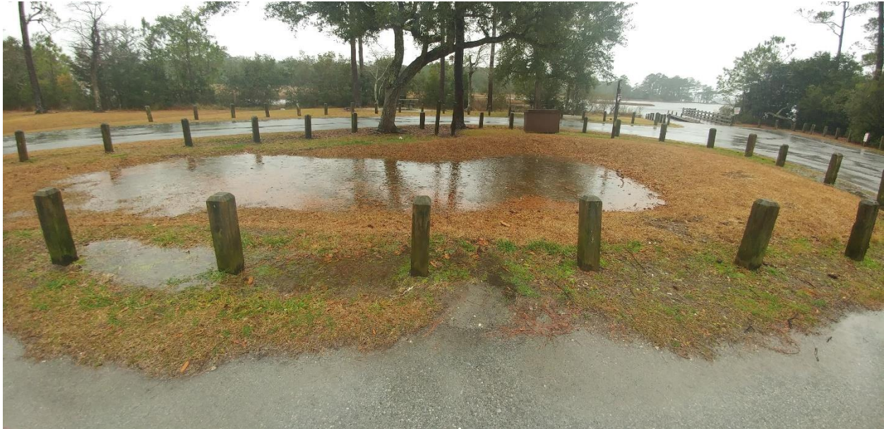
Figure 8: Bio-retention cell at the Cedar Point boat ramp storing runoff after a rain event.
