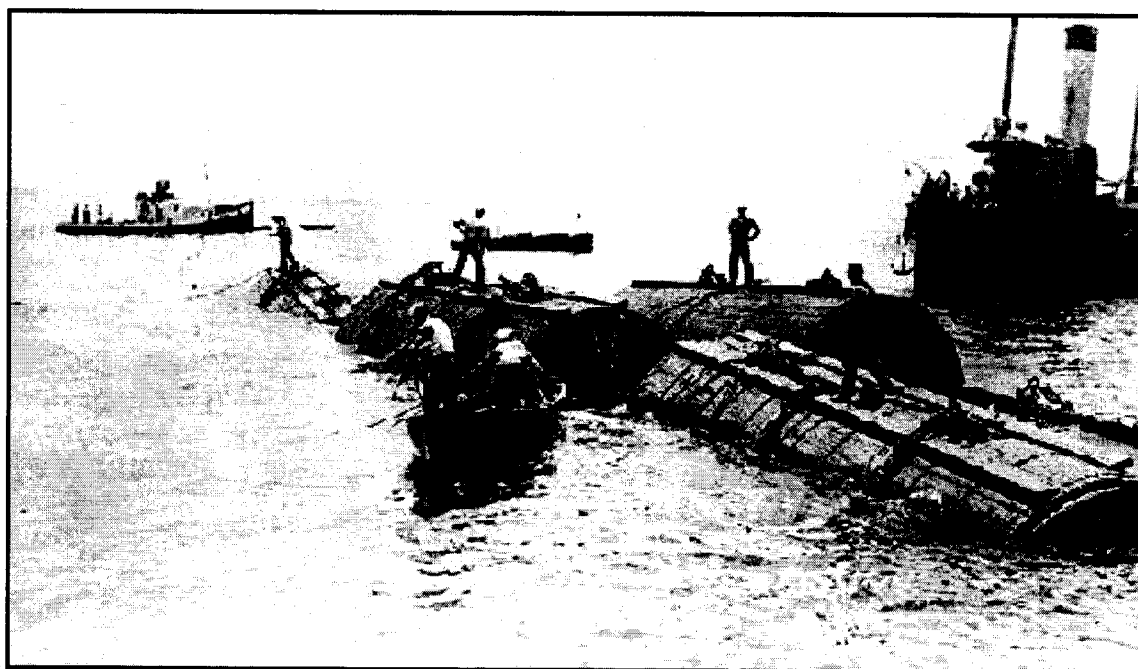
Figure 9. Photo taken of typical salvage pontoons, March 25, 1915, during the recovery of USS F-4 ( www.rddesigns.com ).
